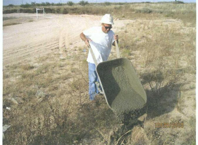
Plugging the monitor well with 1-3% bentonite, concrete slurry
