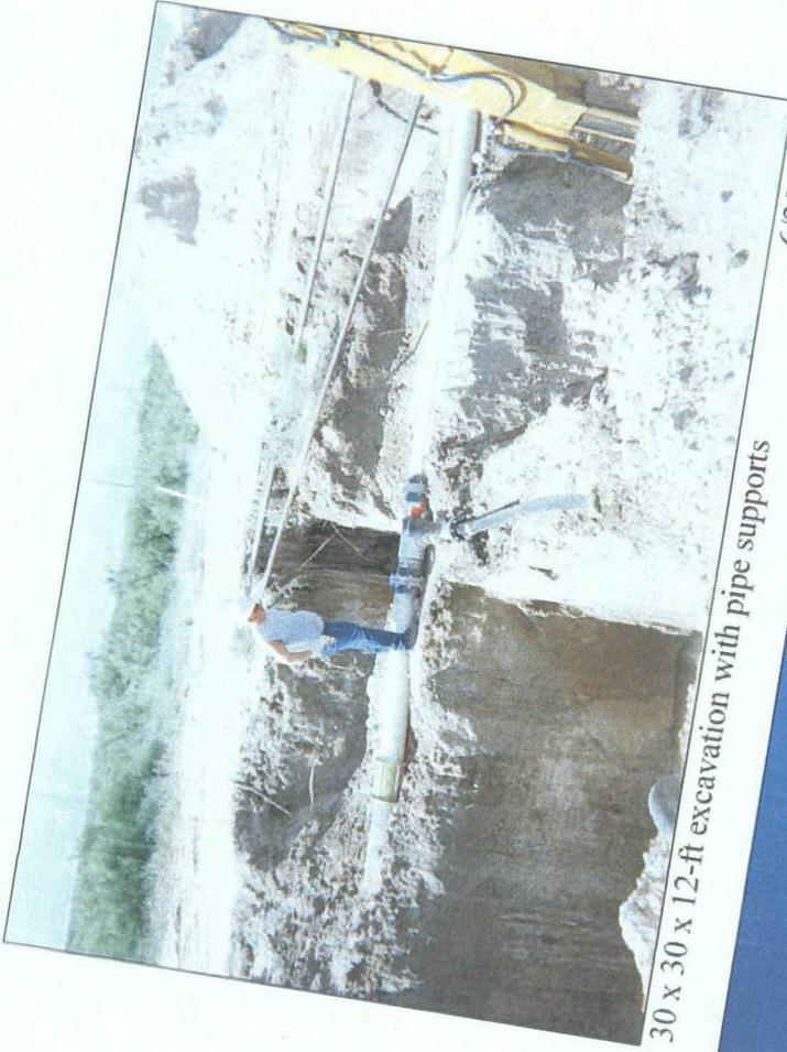
30 x 30 x 12-ft excavation with pipe supports
