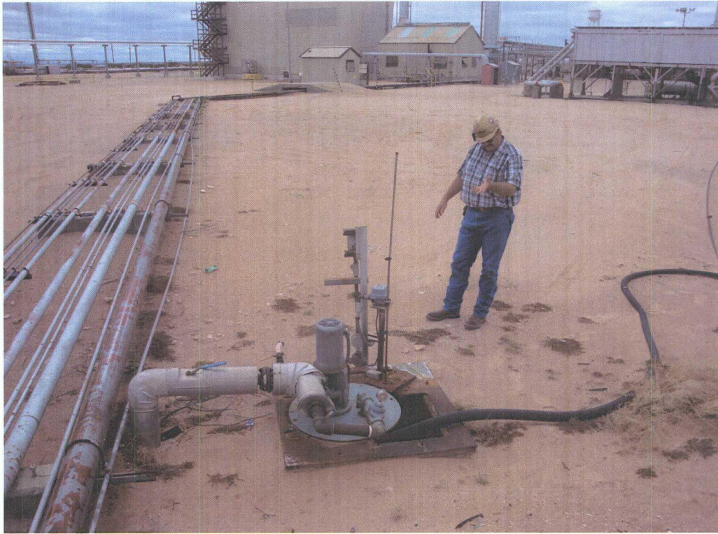
Figure 7: Existing Below-Grade Tank #2 (East Boiler Sump)
