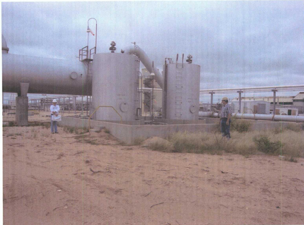
Figure 3: Existing Above-Ground Tanks in Concrete Secondary Containment Which Will Replace Existing Below-Grade Classifier Tanks
