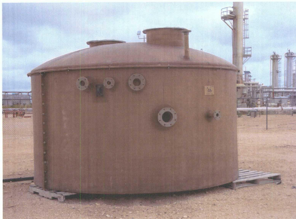
Figure 4: Typical Fiberglass Double-Walled Below-Grade Tank
