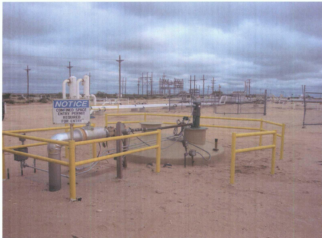
Figure 6: Completed New Below-Grade Tank "West Sump" Installation
