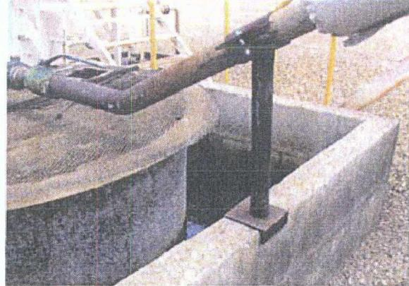
Photo 13: Fluids in secondary containment.
