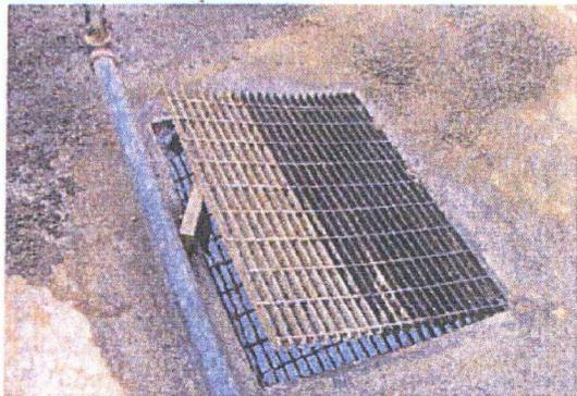
Photo 2: Sump in secondary containment used as a below grade tank.
