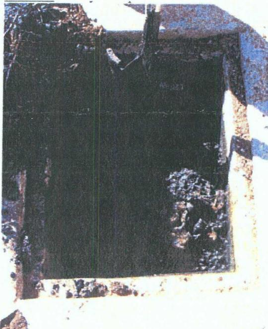
Photo 3: No drainage within sump.
