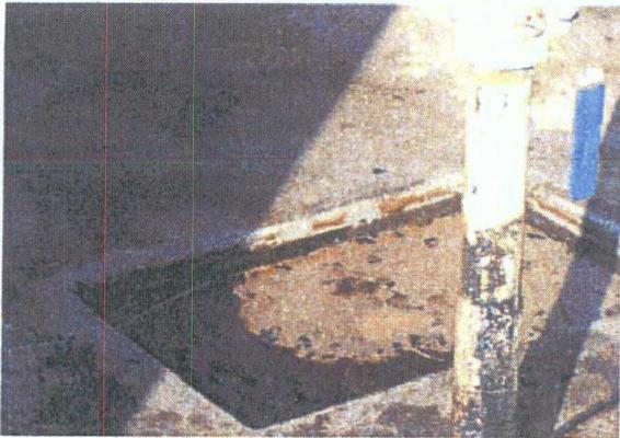
Photo 1: Sump being used as a below grade tank.
