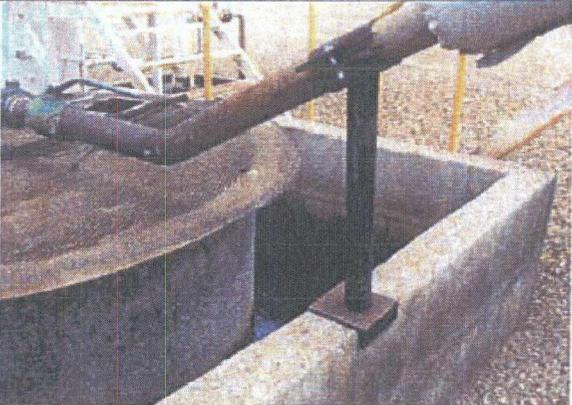
Photo 13: Fluids in secondary containment.
