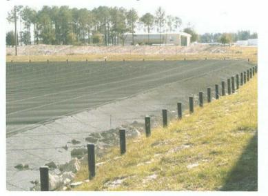
This system has proven to withstand snow and wind loads while effectively hiding the water surface from the view of migratory birds. This netting provides considerable shade on the water surface and will hinder evaporation to some extent.
