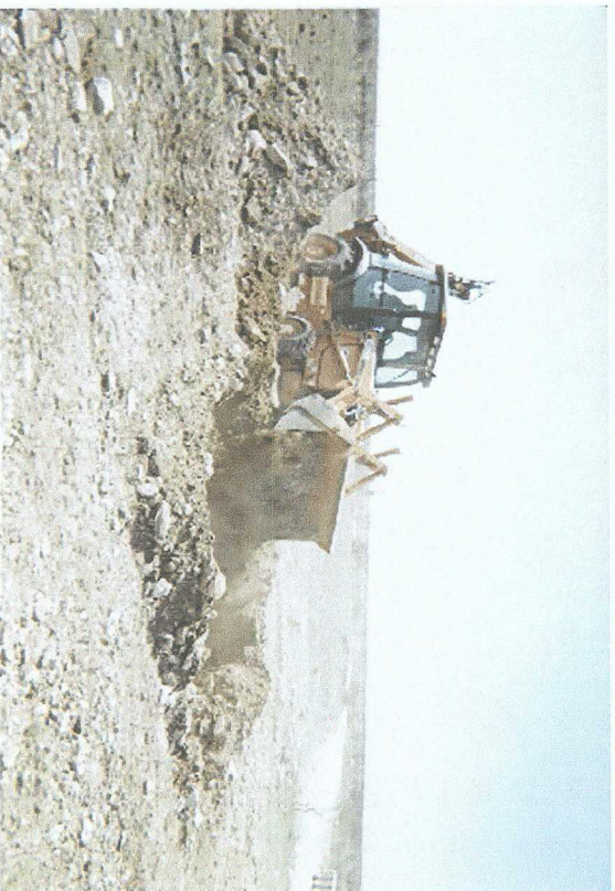
Backfilling excavation
