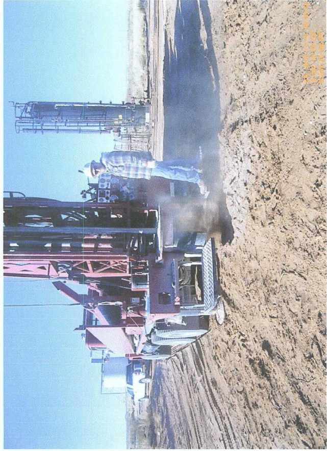
Installing Soil Bore
