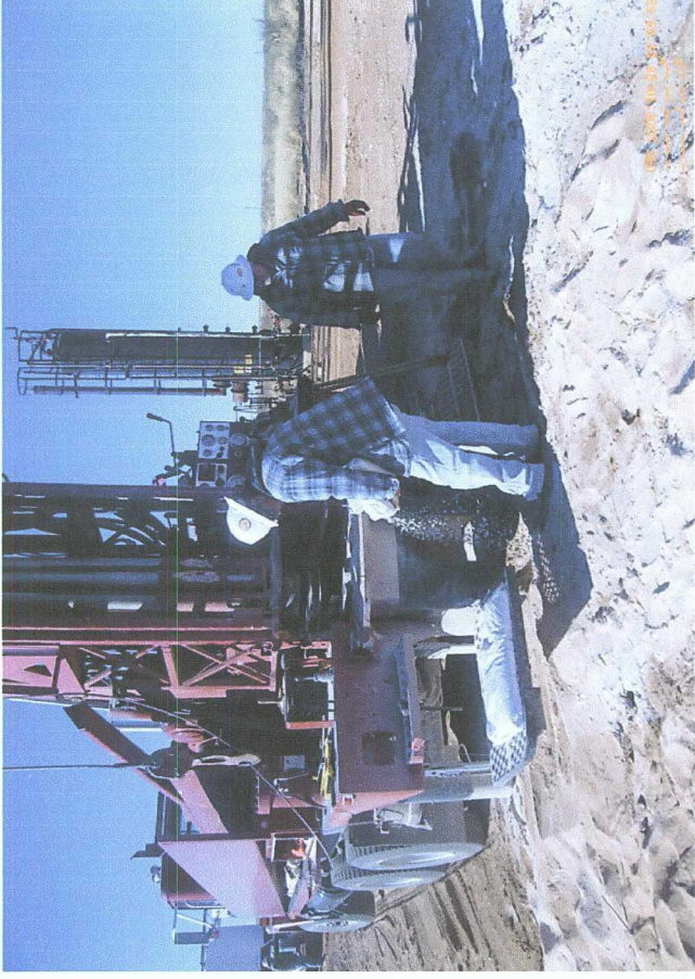
Plugging the soil bore with bentonite
