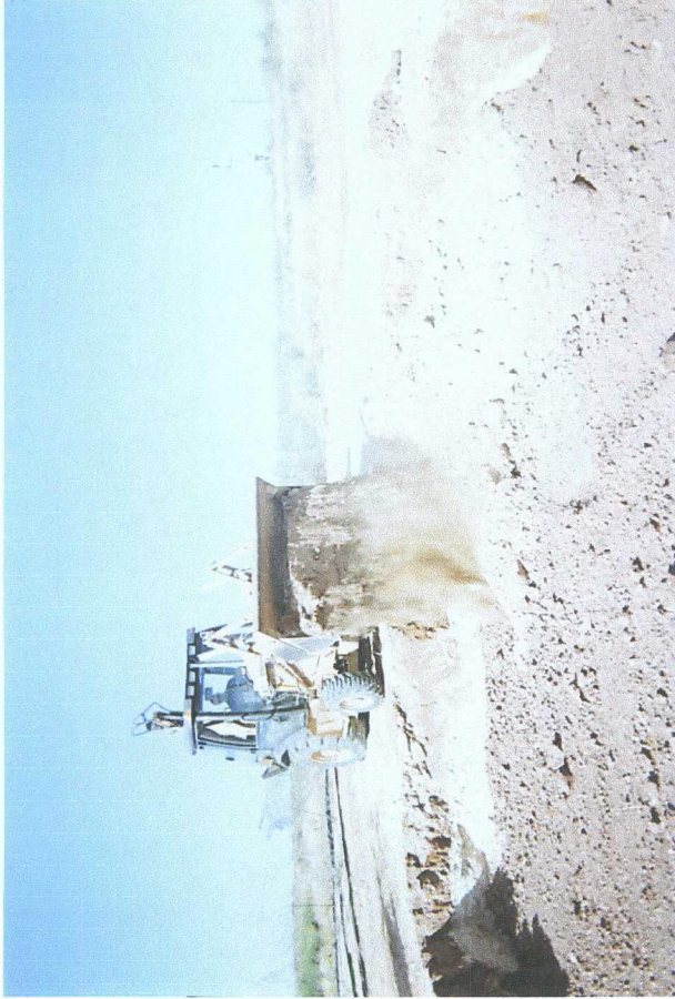
Backfilling excavation above clay liner
