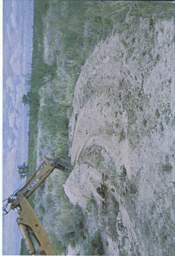
Backfilling excavation
