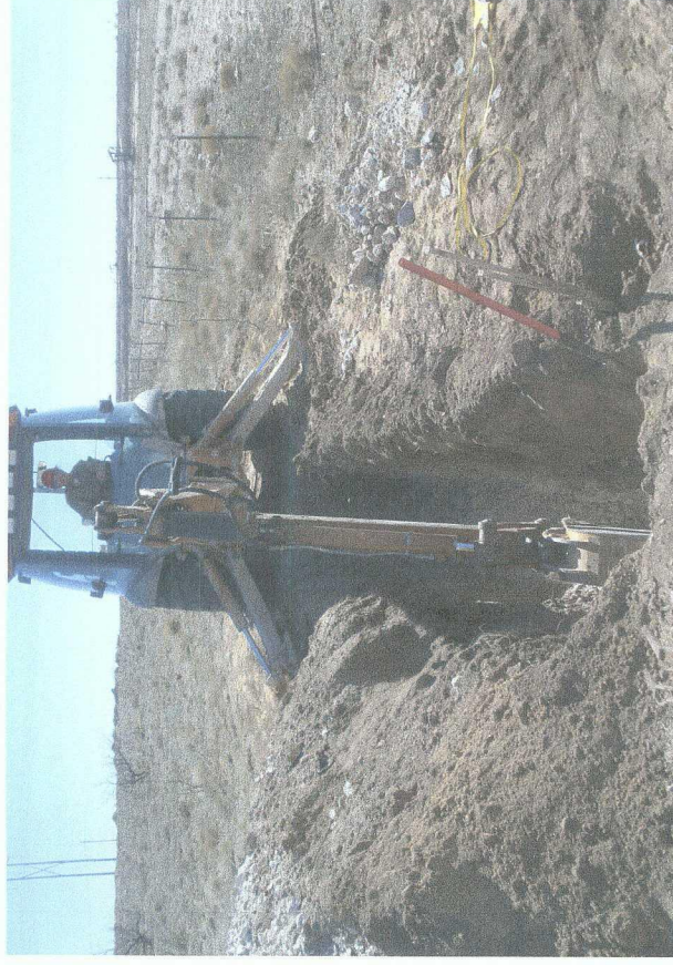
Delineation trench being excavated
