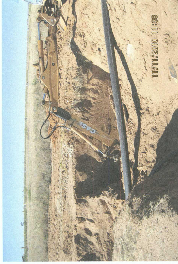
Delineation trench being excavated
