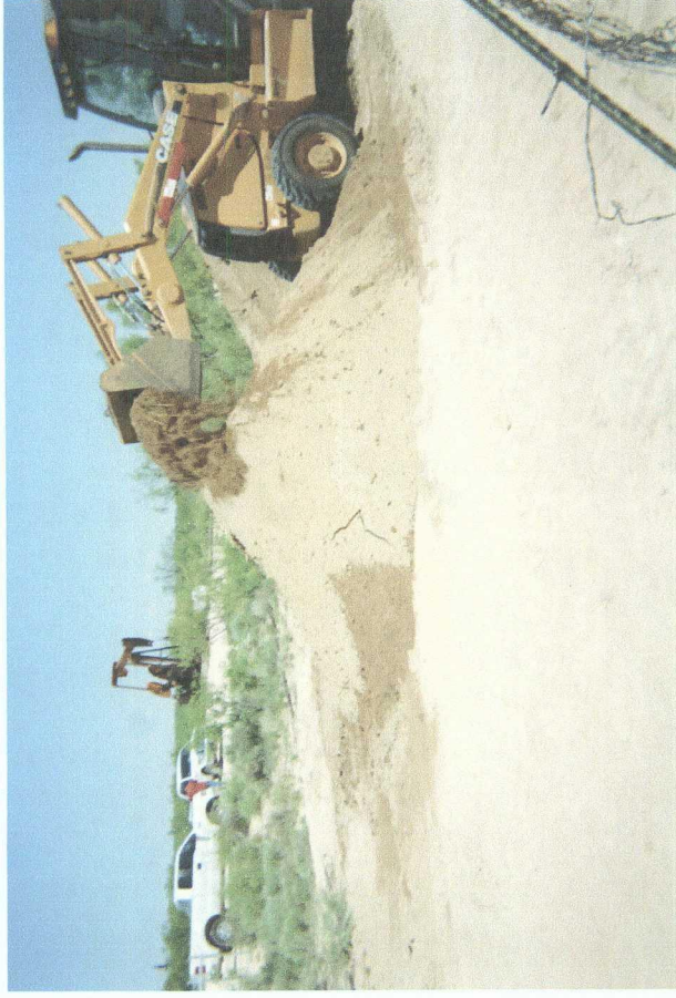
Blending backfill with clean imported soil
