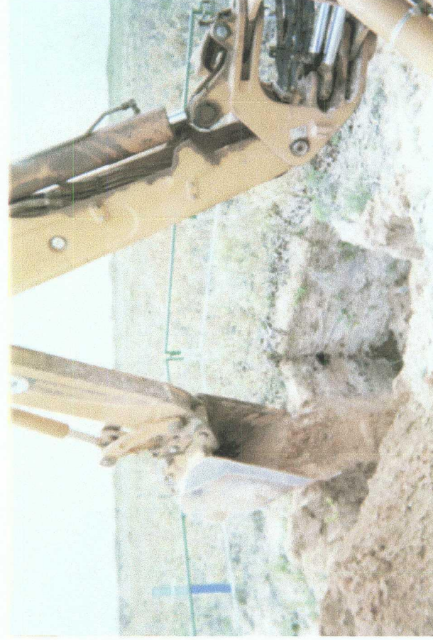
Backfilling excavation
