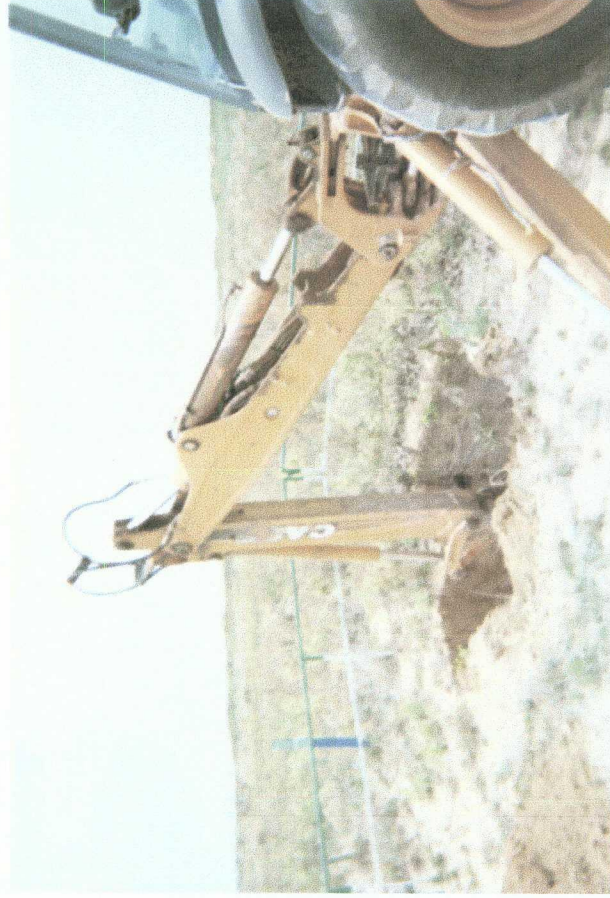
Delineation trench being excavated
