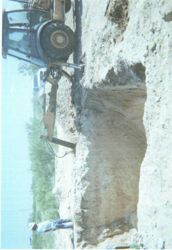
Delineation trench being excavated
