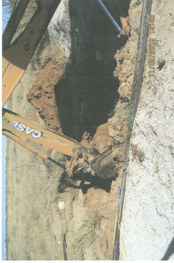
Delineation trench being excavated
