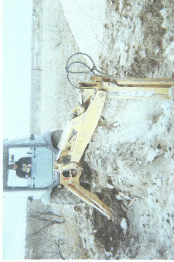
Delineation trench being excavated
