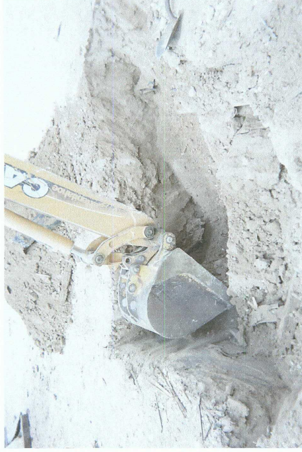
Delineation trench being excavated
