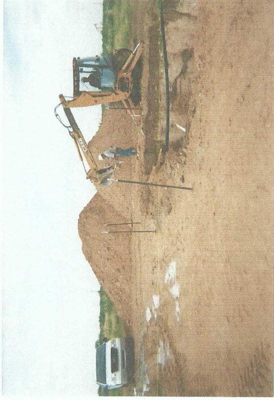
Delineation trench being excavated
