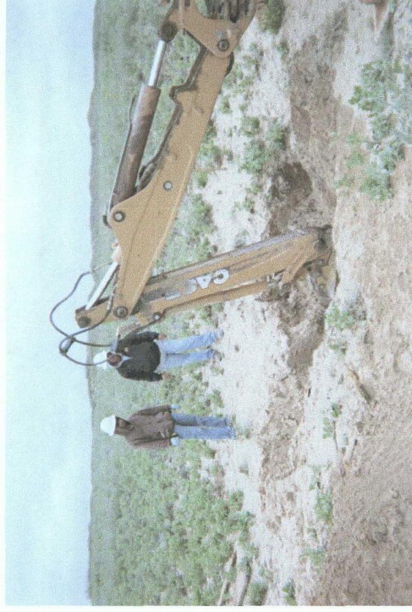
Delineation trench being excavated
