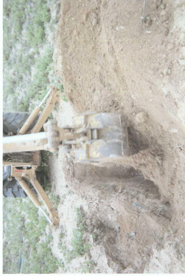
Backfilling excavation
