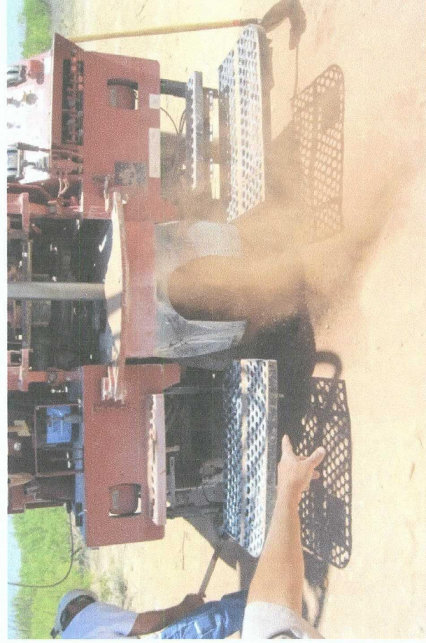
Drilling the bore hole 5/13/10
