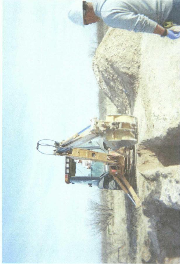
Delineation trench being excavated
