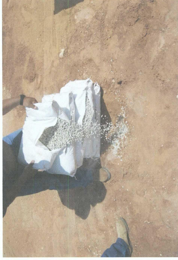
Plugging the bore hole with Bentonite 5/18/10
