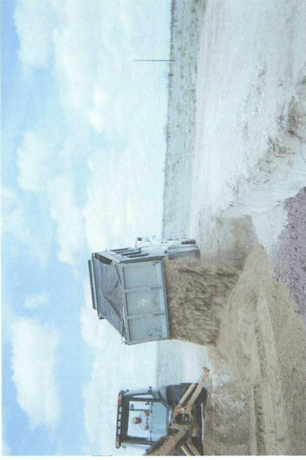
Backfilling above clay barrier with imported soil
