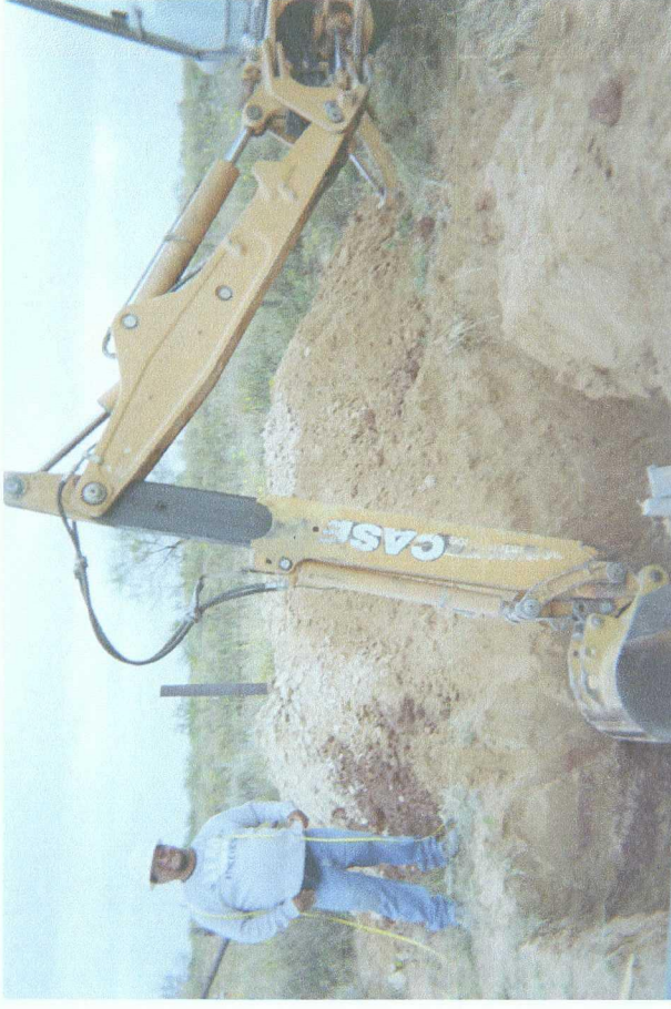
Delineation trench being excavated
