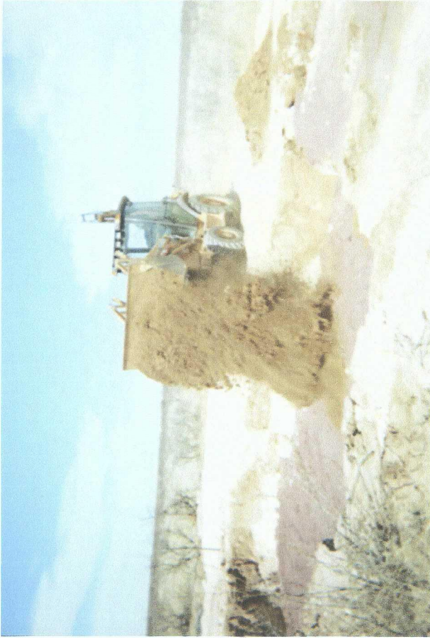
Backfilling excavation above clay liner
