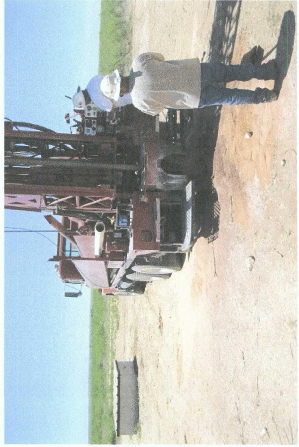
Drilling the soil bore
