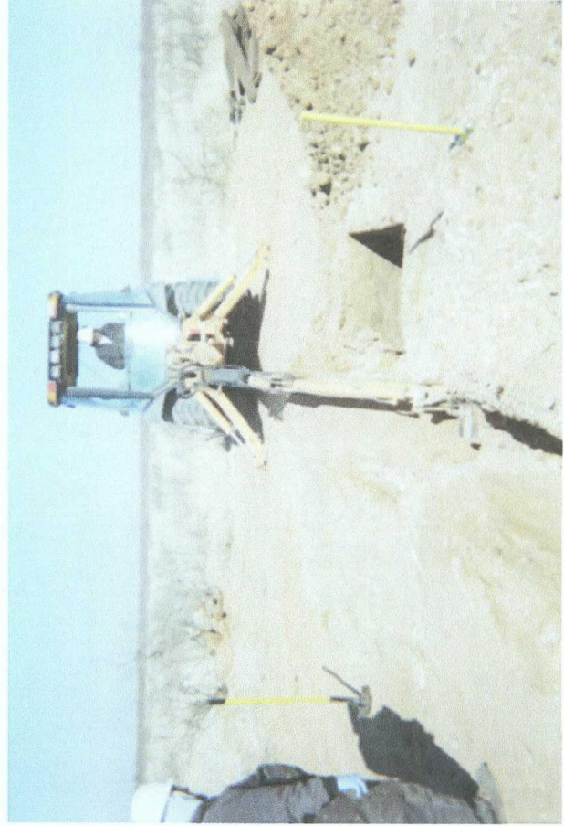
Delineation trench being excavated
