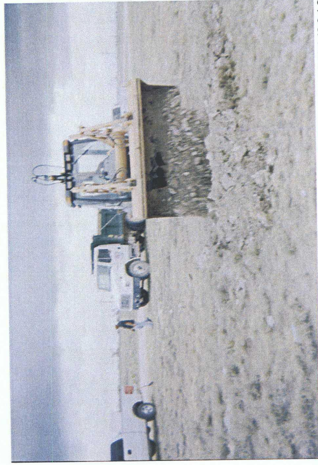
Backfilling excavation
