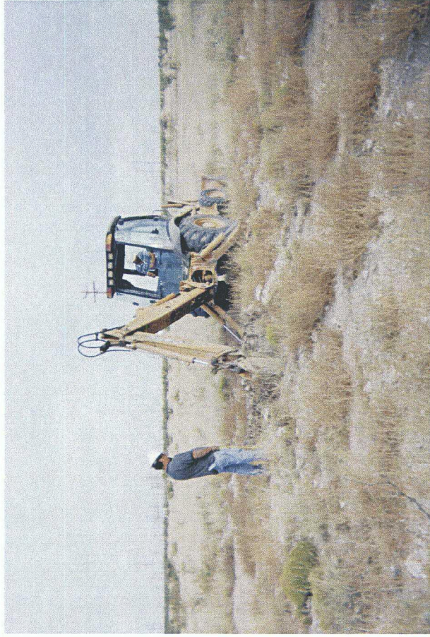
Digging initial vertical delineation trench
