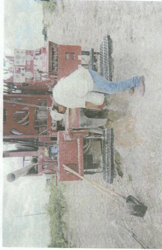
plugging SB #1 with bentonite
