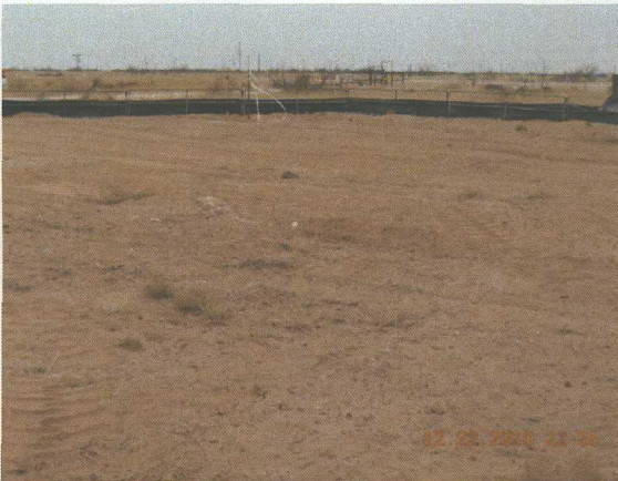
Completed the spreading of the top soil and peanut hay
