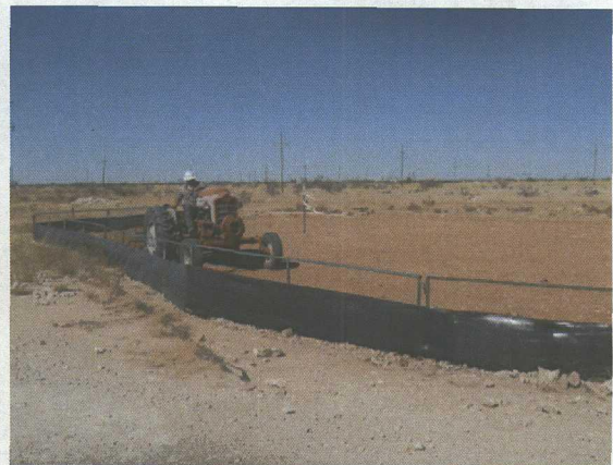
Discing the site for seeding (2-15-11)
