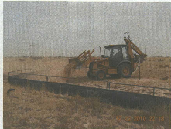
Spreading the top soil with peanut hay mix
