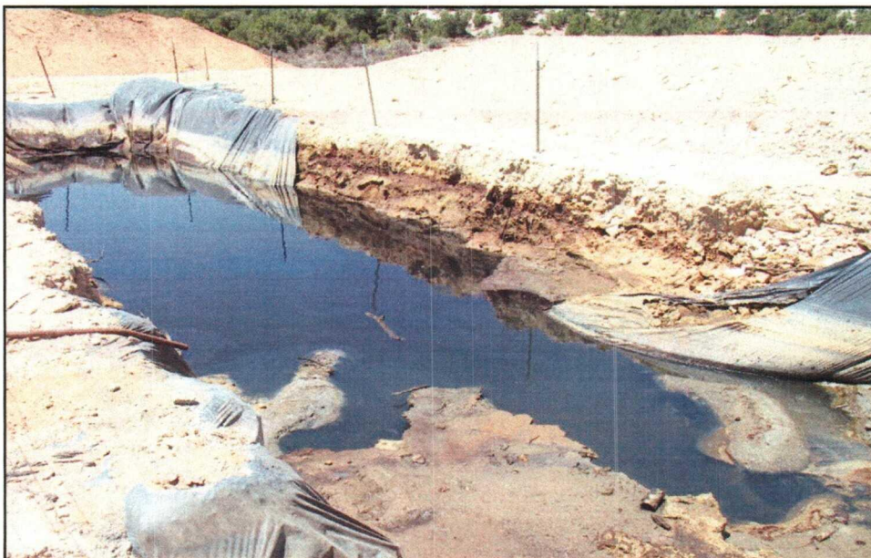
Drilling pit with torn liner
