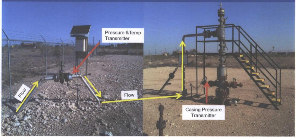
Pressure Transmitters are connected to the casing valve on all injection wells in NHU
