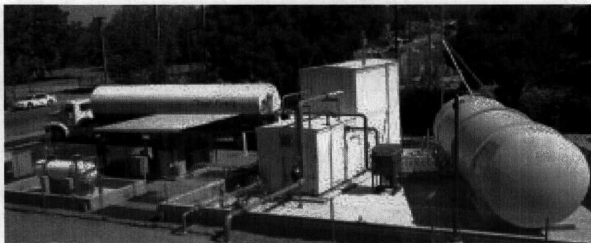
Figure 8 .Idaho National Labs Small Scale Natural Gas Liquefaction Plant and Storage Tank. This unit is shown to indicate the compact nature of the technology.
