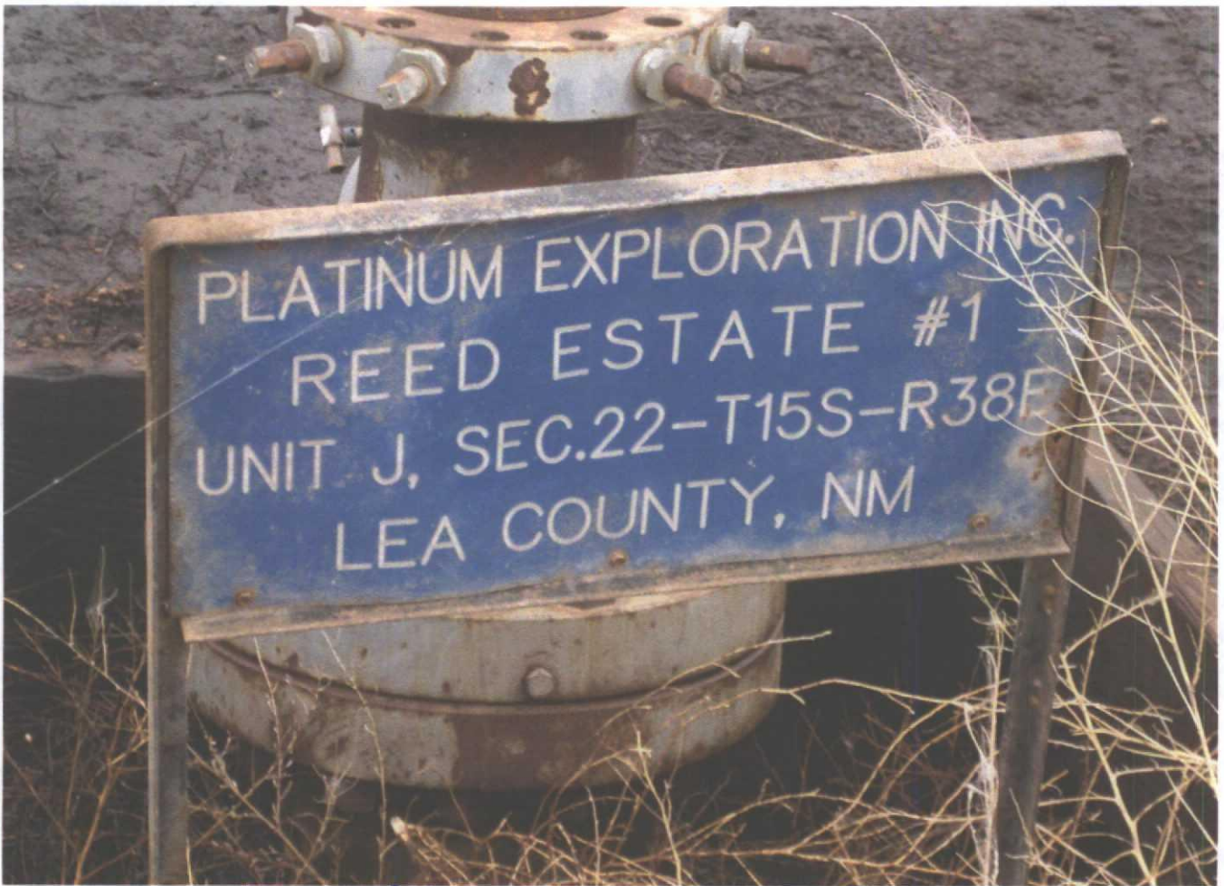
WRONG OPER. ON SIGN ↑ 30-025-07258
