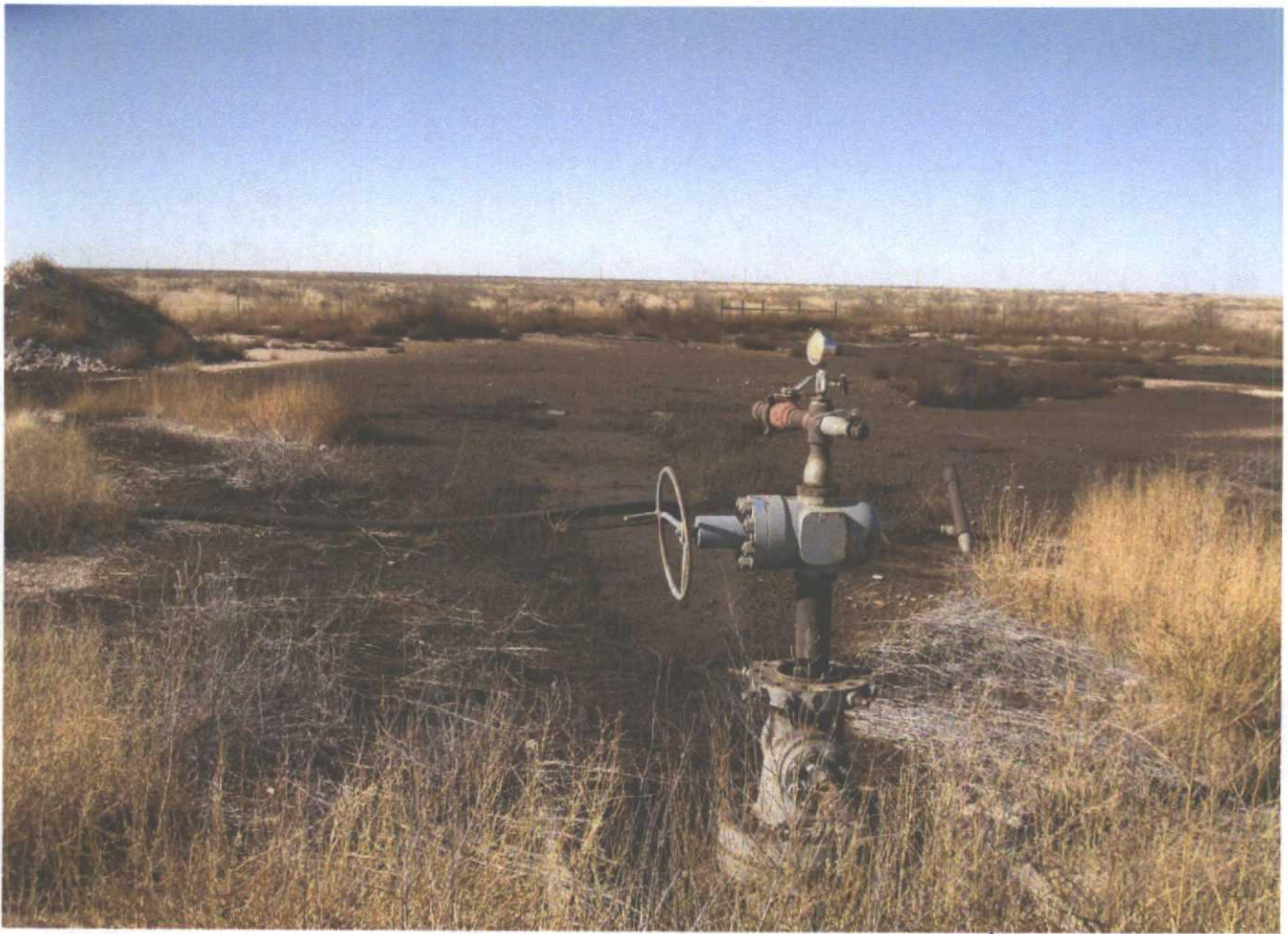
LOOKING FROM SE TO NW
