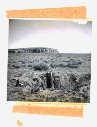
ONE OF TWO HOLES IN SW/4 NE/4 SEC. 2, T. 20 N., R. 30 E., Harding County, N.M., showing derrick foundation and protruding pipe. Hole is plugged with wood, presumably fence post. No indication of cement plug at surface. Annulus open to atmosphere. Pits open but not dangerous to livestock due to erosion over the years. Location not cleared. Camera at approximately 50 feet, looking to eastward. This hole is presumably Tixier No. 1.
