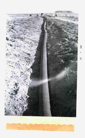
VIEW LOOKING SOUTHEAST FROM TIMMONS CARBONIC CO. PLANT TO NEW WELL drilled recently at a distance of 1/h mile. View shows "invasion pipe" flow lines employed in this area. In this case, the entire flow line from well to plant consisted of this rubber impregnated fabric. In the case of the Timmons No. 1 well, approximately 75 feet of the 1/2 mile line consists of this type pipe.
