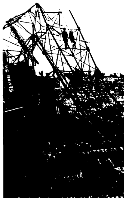
Collapsed rig on wildcat well 11 1/2 miles northeast of the Hospah field, 1927. (Photo courtesy of Tom Dugan)
