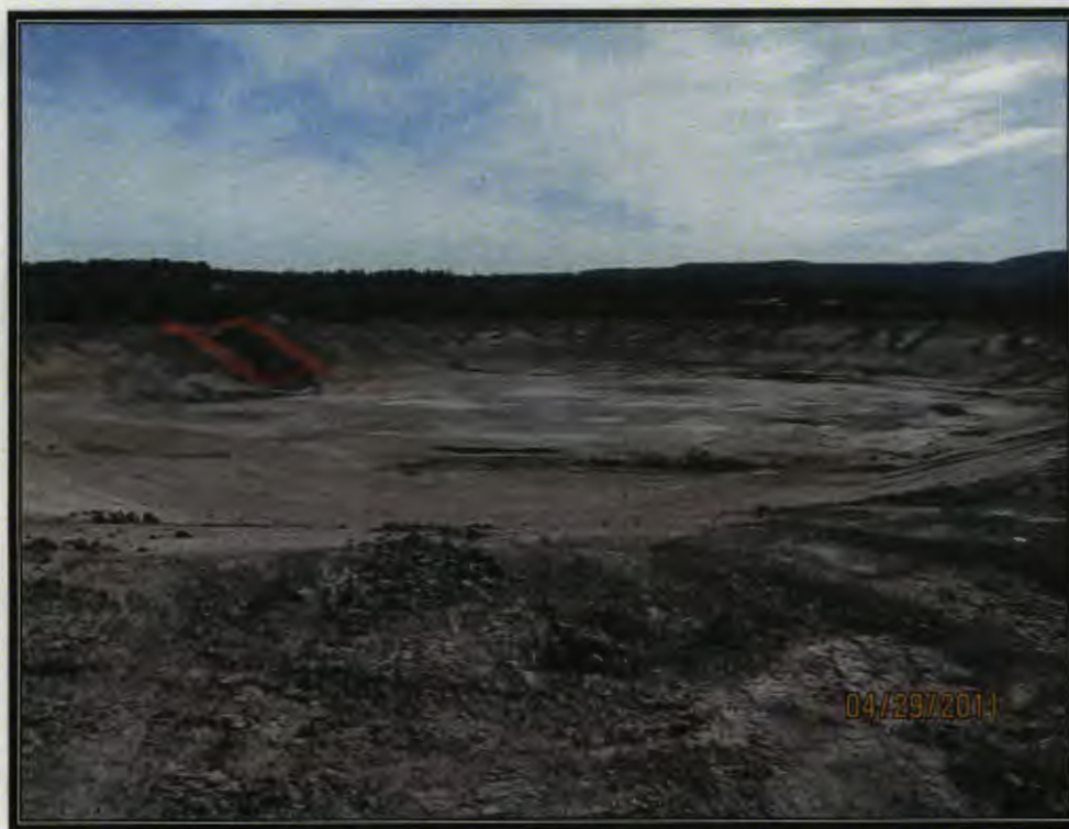
Photo 6: Pond after Liner and Leak Detection Removed
