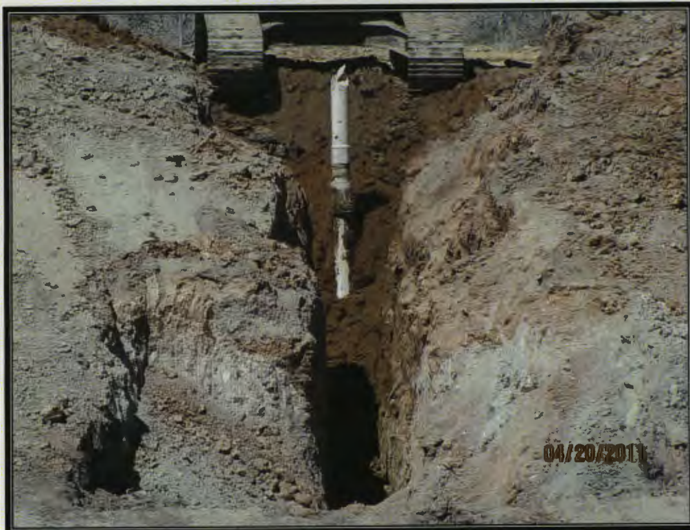
Photo 4: Removing the Leak Detection System
