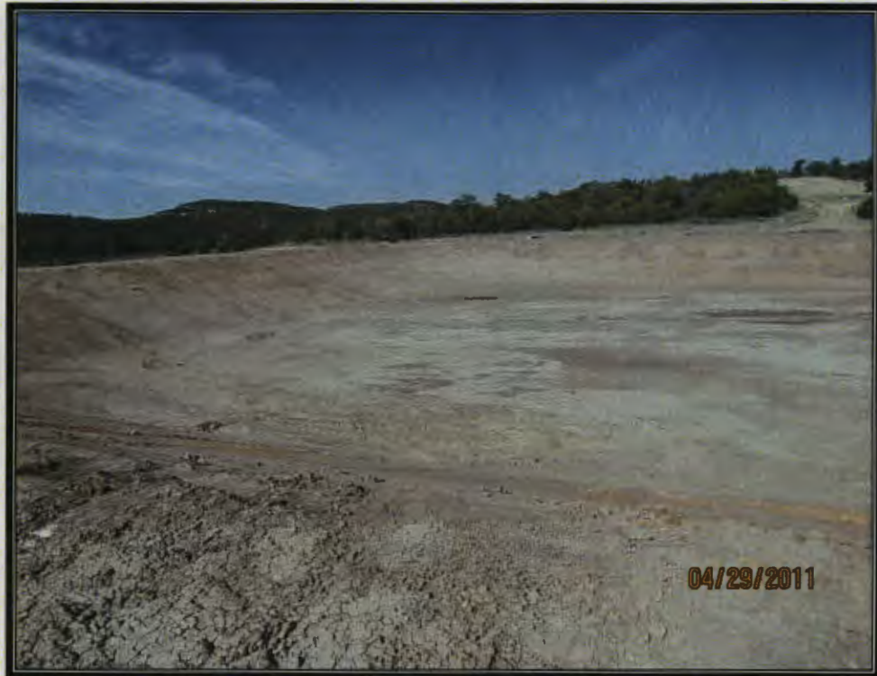
Photo 7: Pond after Liner and Leak Detection Removed
