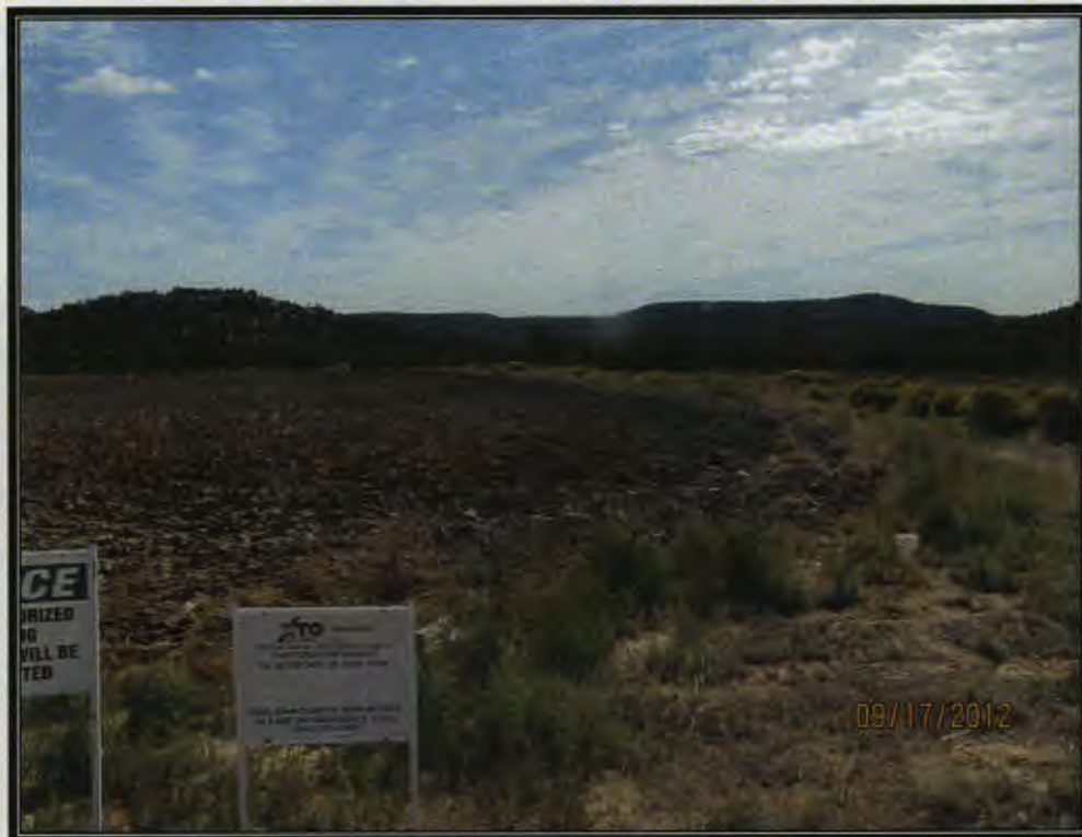
Photo 9: Pond after Backfill and Reclamation (View 1)
