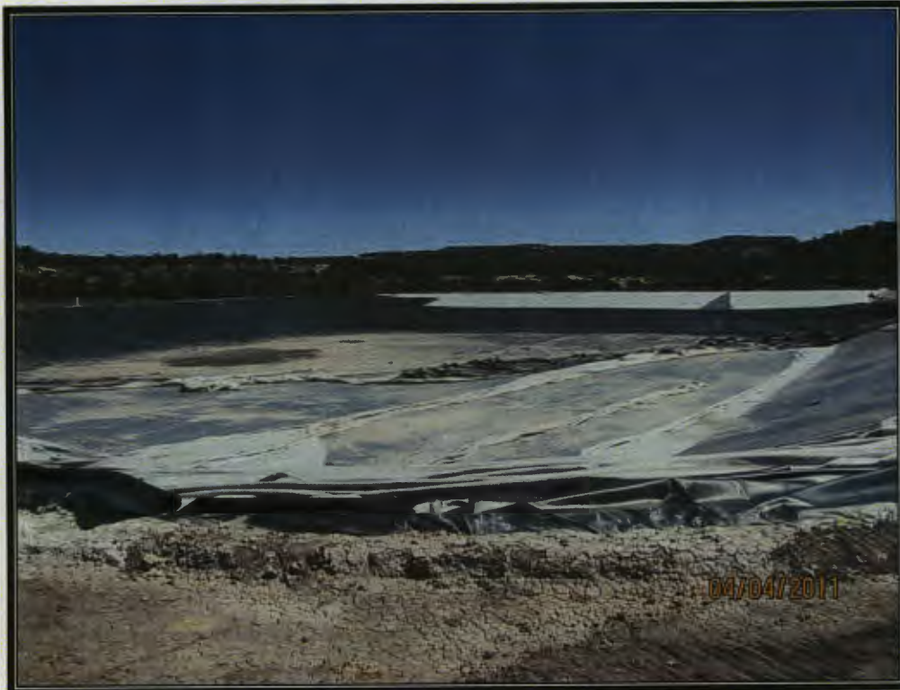
Photo 3: Removing the Liner
