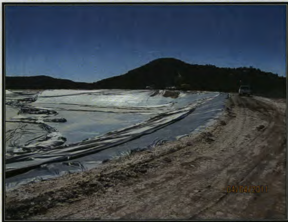
Photo 2: Removing the Liner
