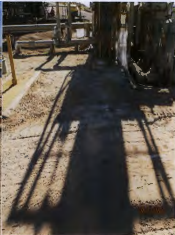
North-east side of the benzene strippers
