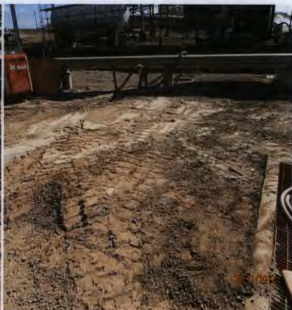
East side of the benzene strippers
