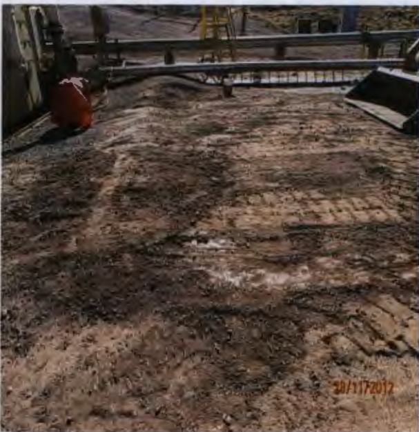
West side of the benzene strippers
