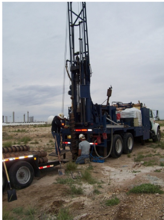
No. 10 – View looking northeast at an 8'' HSA advancing a soil boring; boring was completed into MW-06.
