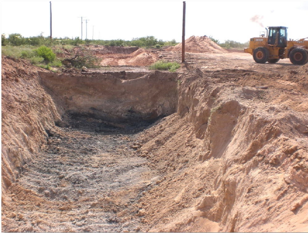
No. 25 – View looking west at excavation east of power poles; note discolored soils in bottom of excavation.
