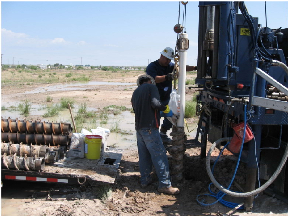
No. 16 – Installing 4" diameter PVC in MW-06.
