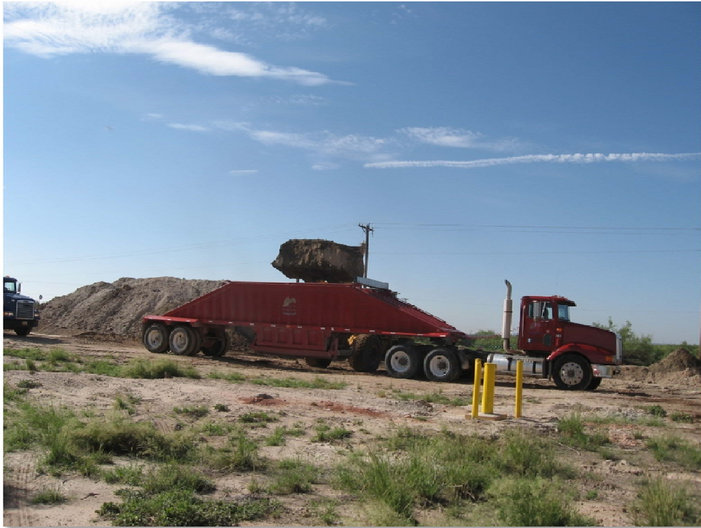
No. 27 – View of loading of contaminated soil into 20 cubic yard belly dump hauler. Note MW-06 in foreground.
