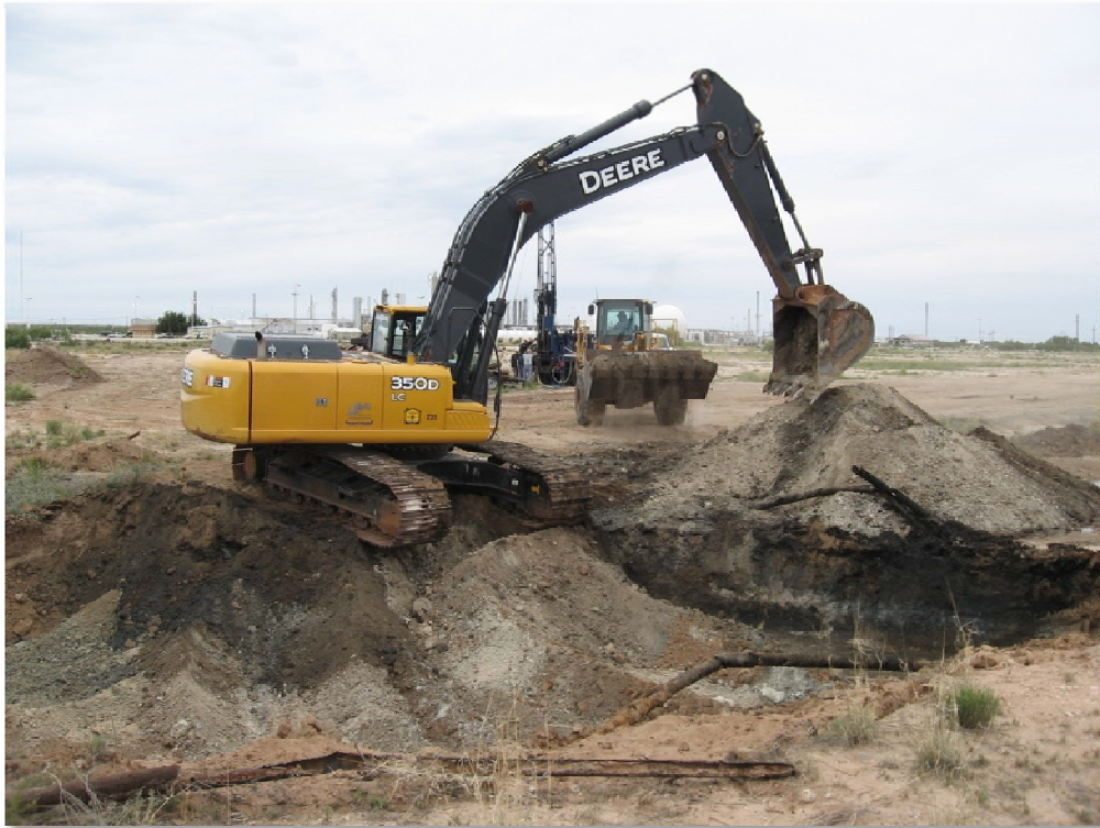
No. 21 – View looking north at trackhoe excavating pit; note metal pipe in pit.
