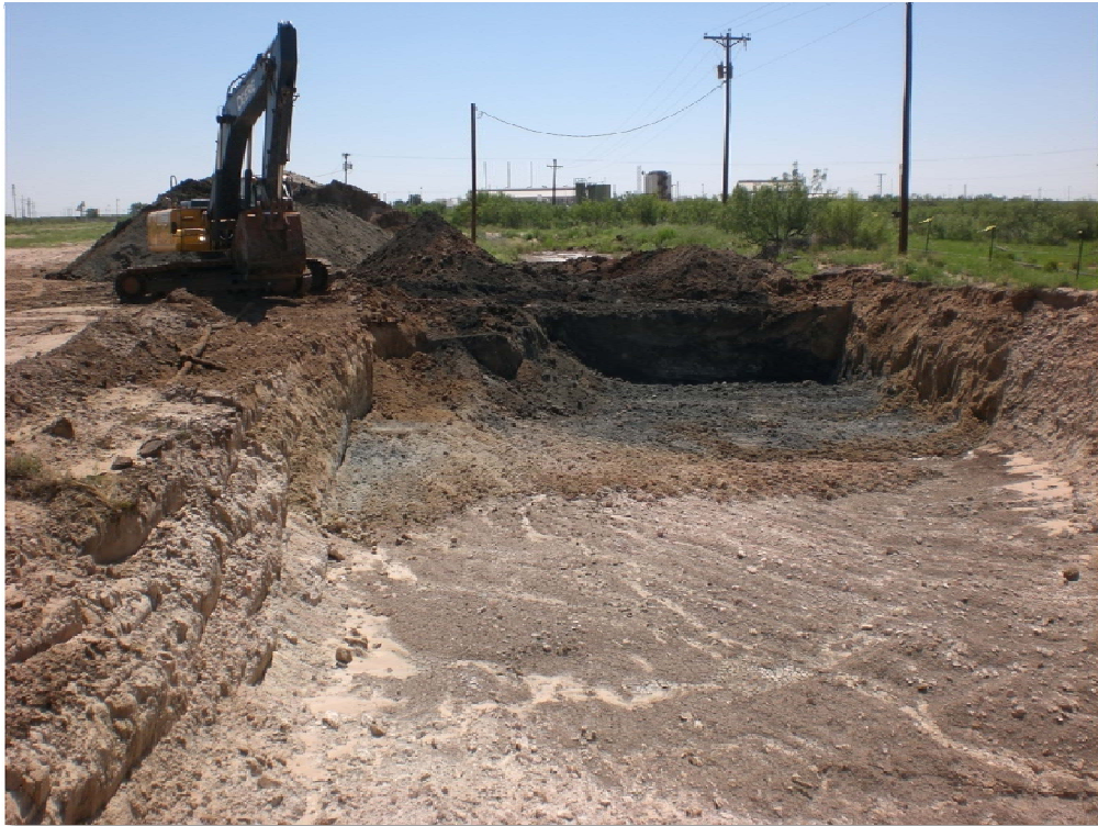
No. 19 – View looking east at excavated pit and track hoe used for excavation. Note stockpiled soils in background, berms around pit and stockpiled soil, and dark soils south of trackhoe.
