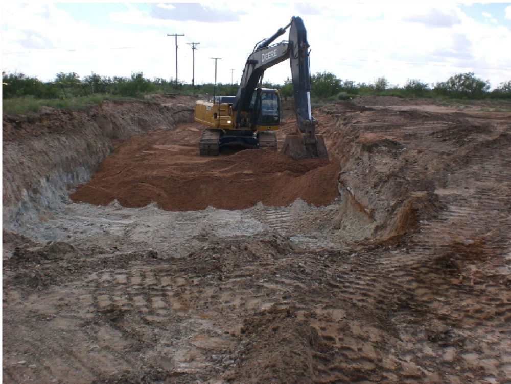
No.22 – View looking west at track hoe compacting backfill material.
