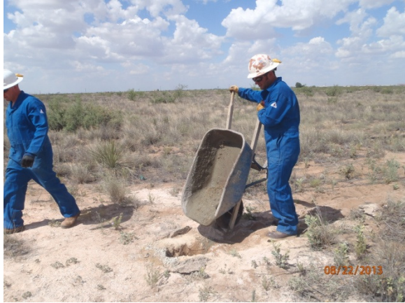
Plugging MW-2 with a 1-3% bentonite/concrete slurry with a 3 ft concrete cap, facing north 8/22/13
