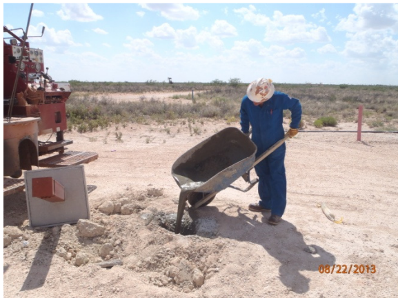
Plug MW-1 with a 1-3% bentonite/concrete slurry and a 3 ft concrete cap, facing west 8/22/13
