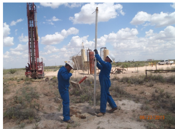
Removing PVC pipe from MW-2, facing southeast 8/22/13
