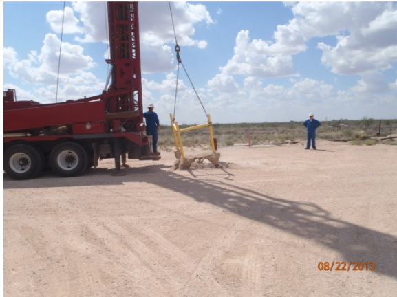
Removing MW-1 guard rail, facing west 8/22/13
