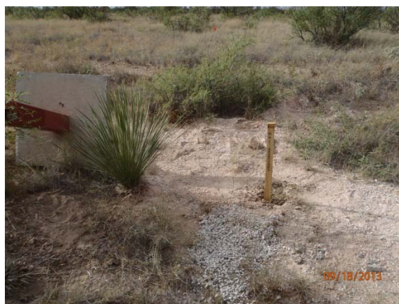
MW-1 plugged and abandoned, facing south 9/18/13
