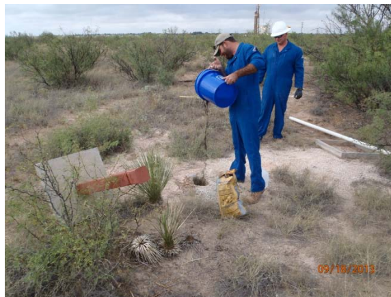
Backfilling bore with a 1-3% bentonite/concrete slurry and a 3 ft concrete cap, facing southwest 9/18/13
