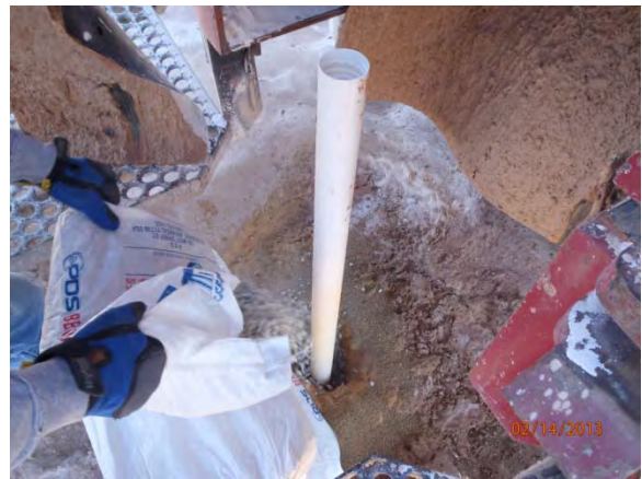
Installing the bentonite seal, facing south 2/14/13
