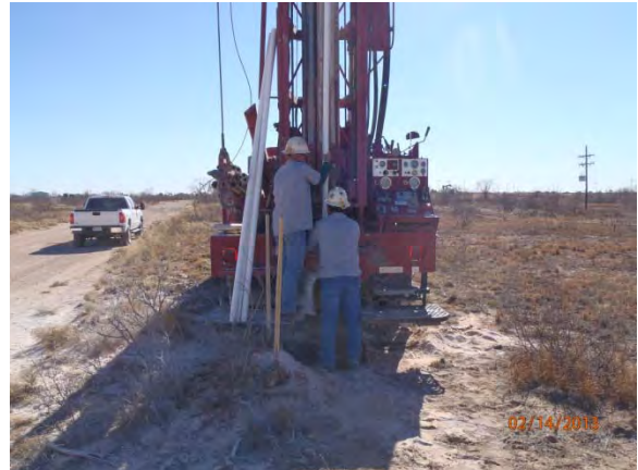
Installing the casing in MW-2, facing south 2/14/13
