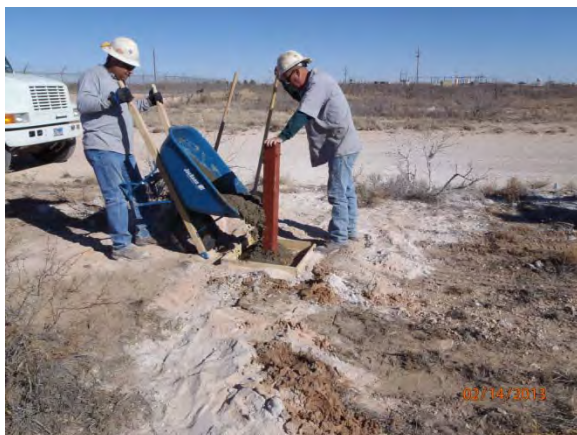
Concreting the well in, facing east 2/14/13
