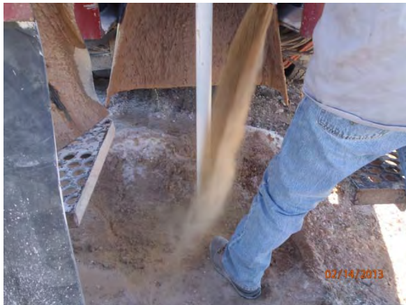
Installing the sand pack, facing south 2/14/13
