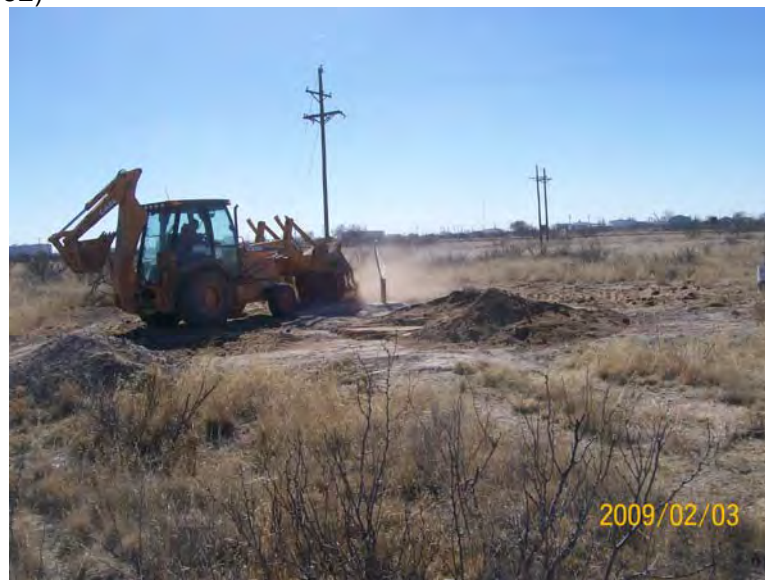
Spreading imported topsoil
