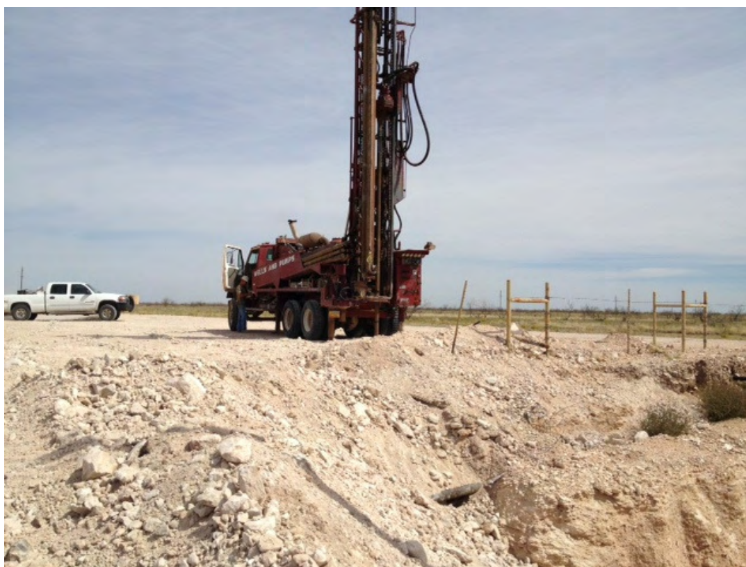
Photograph of the advancement of soil bores at the WLSU #11 remediation site.
