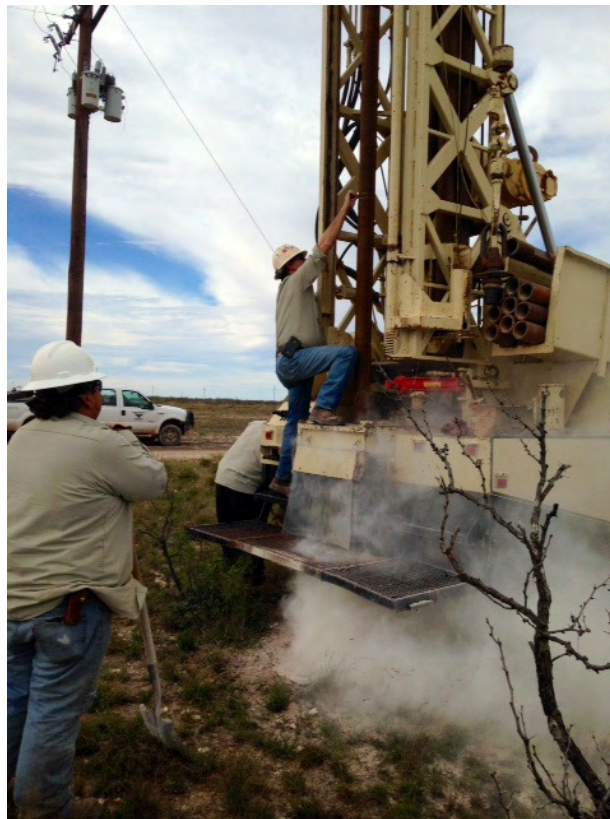
Photograph of the installation of the groundwater monitoring well at the WLSU #11 remediation site.
