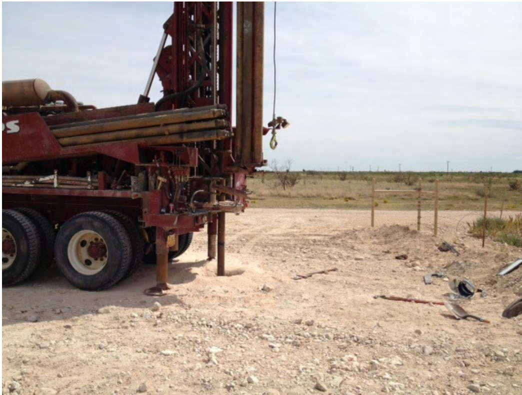
Photograph of the advancement of soil bores at the WLSU #11 remediation site.
