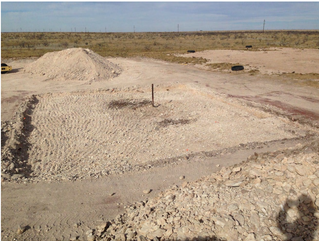
Photograph of the excavated area around the plugged and abandoned well at the WLSU #11 remediation site.
