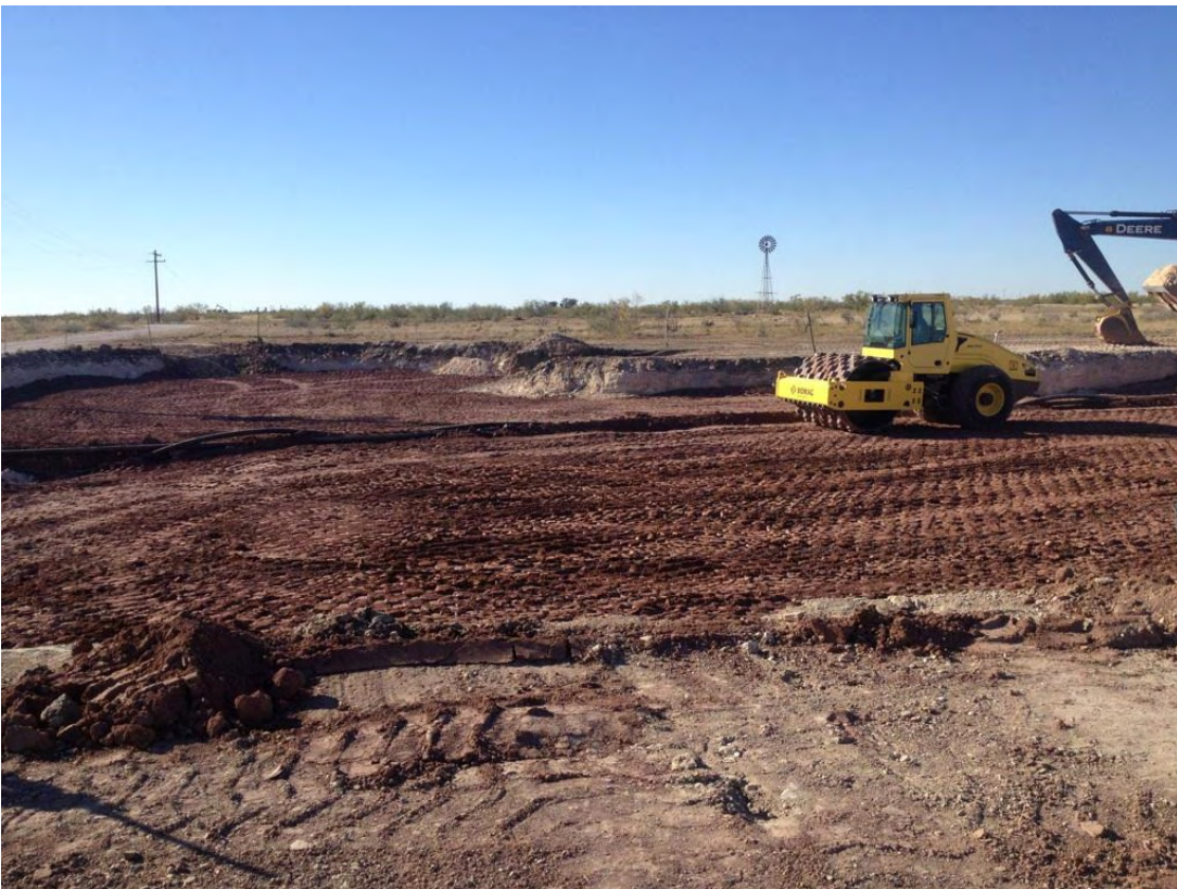
Photograph of the installation of the clay liner at the WLSU #11 remediation site.
