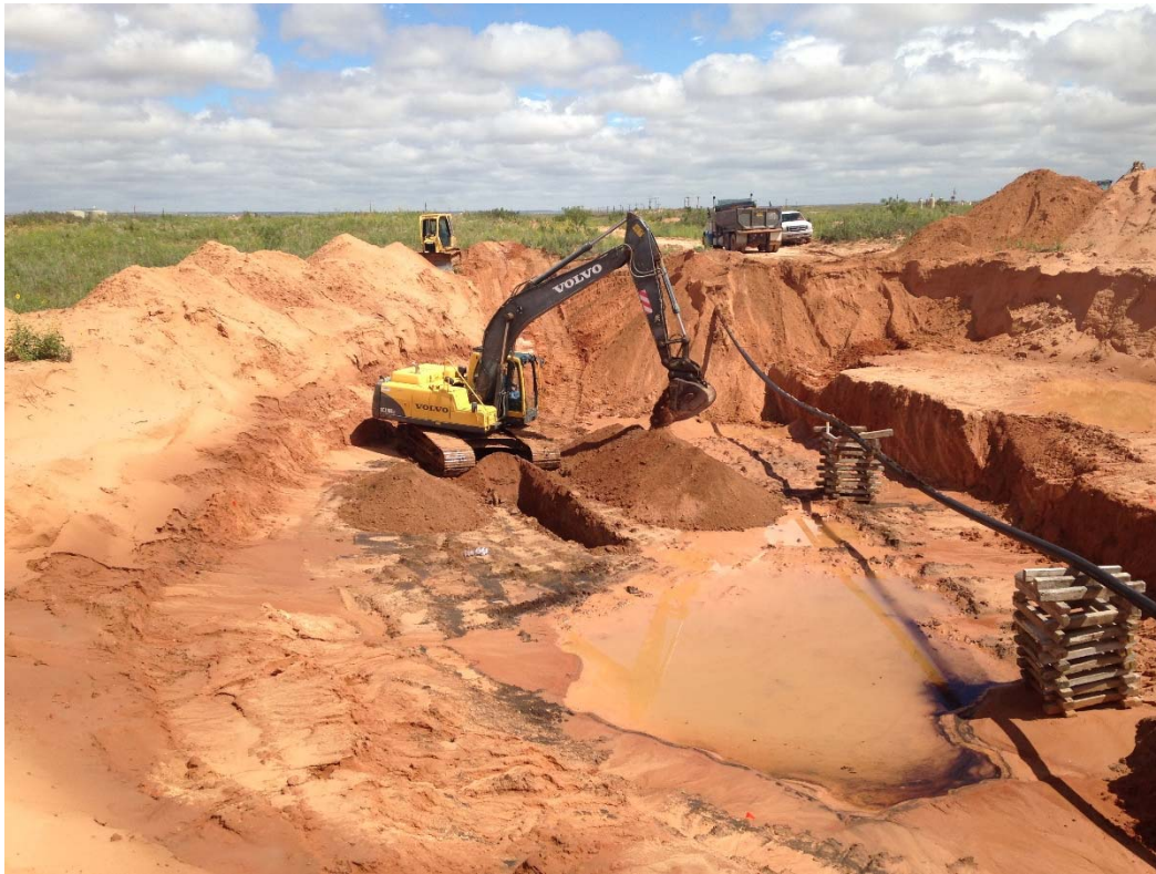
Photograph of the advancement of delineation trench in the Eastern Release excavation at the QPQASU #10 Remediation Site.
