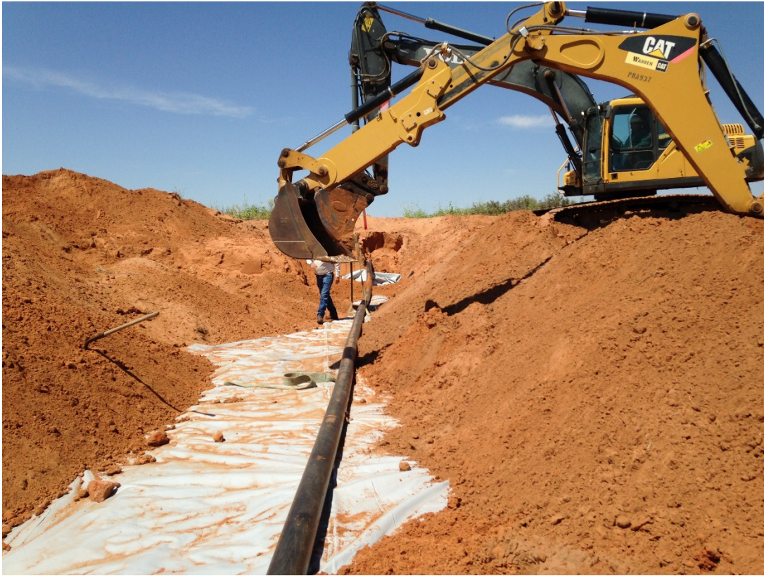
Photograph of backfilling activities related to the Western Release at the QPQASU #10 Flow Line Remediation Site.
