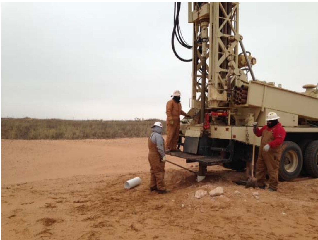
Photograph of the advancement of environmental soil bores at the QPQASU #10 Flow Line Remediation Site.
