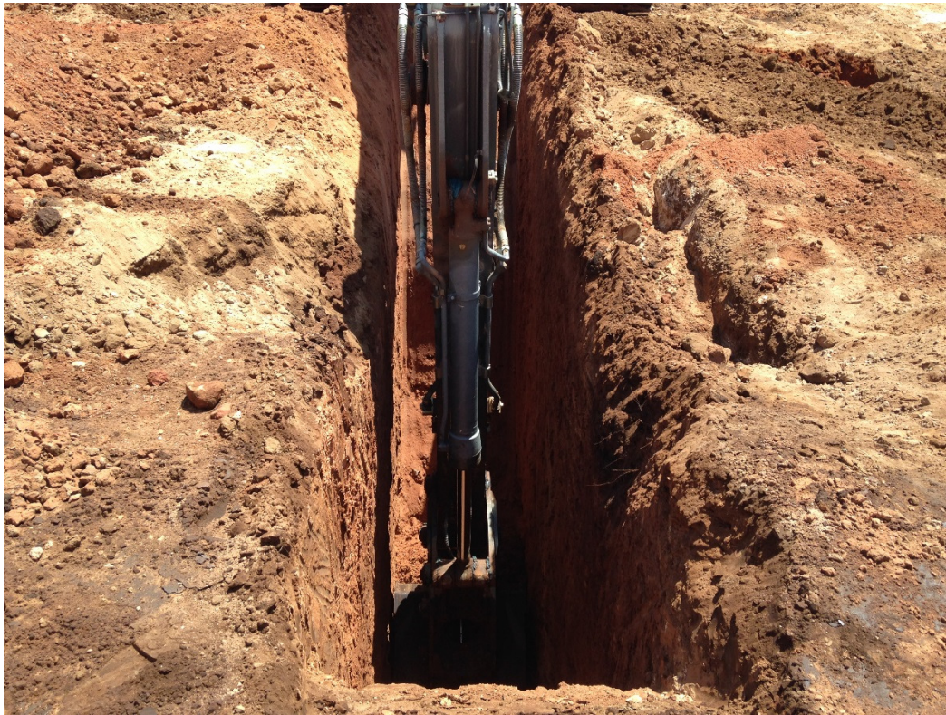
Photograph of the advancement of delineation trench in the Primary Release excavation at the QPQASU #10 Remediation Site.
