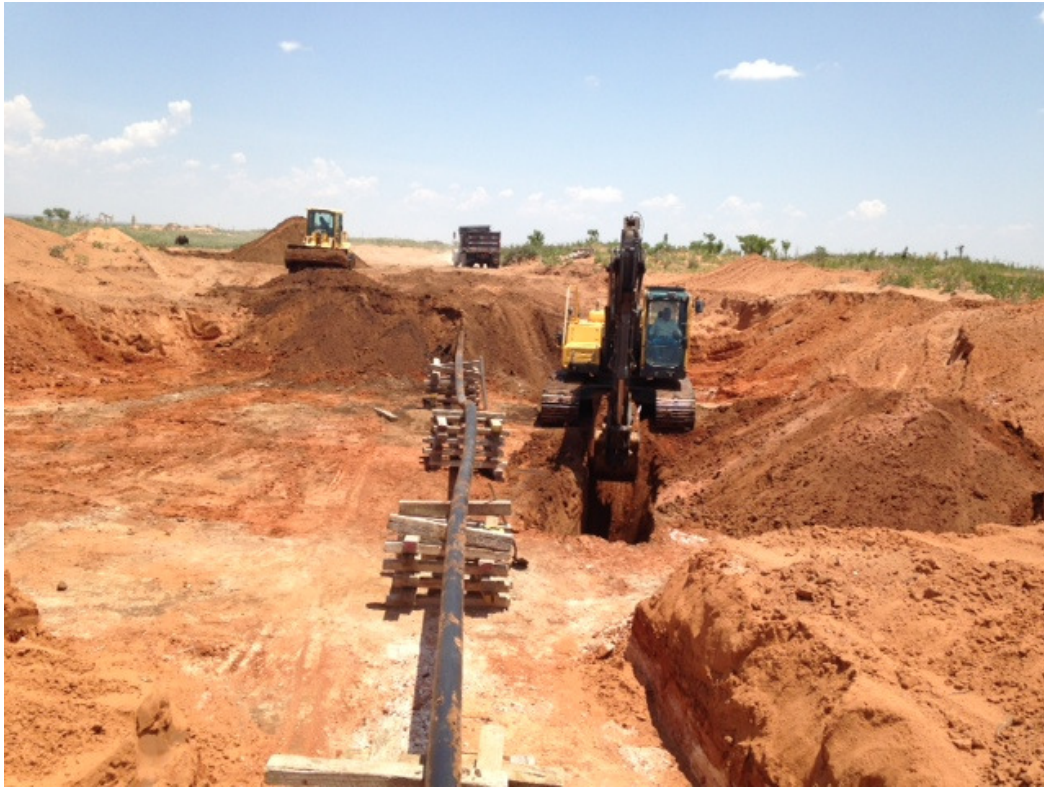
Photograph of the advancement of delineation trench in the Western Release excavation at the QPQASU #10 Remediation Site.
