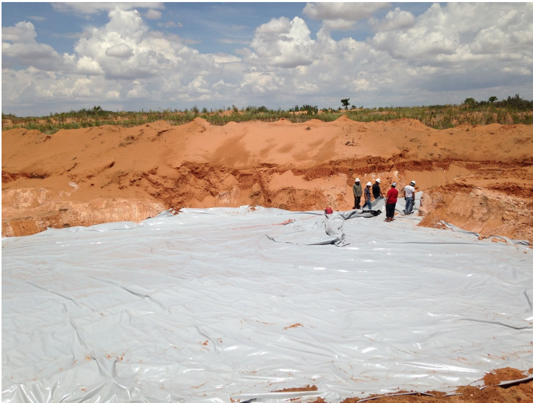
Photograph of the installation of an NMOCD-approved liner in the Primary Release excavation at the QPQASU #10 Remediation Site.
