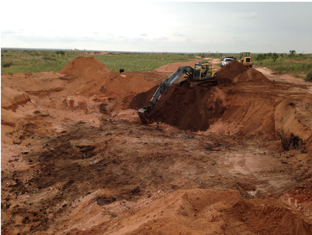
Photograph of excavation activities related to the Primary Release at the QPQASU #10 Flow Line Remediation Site.
