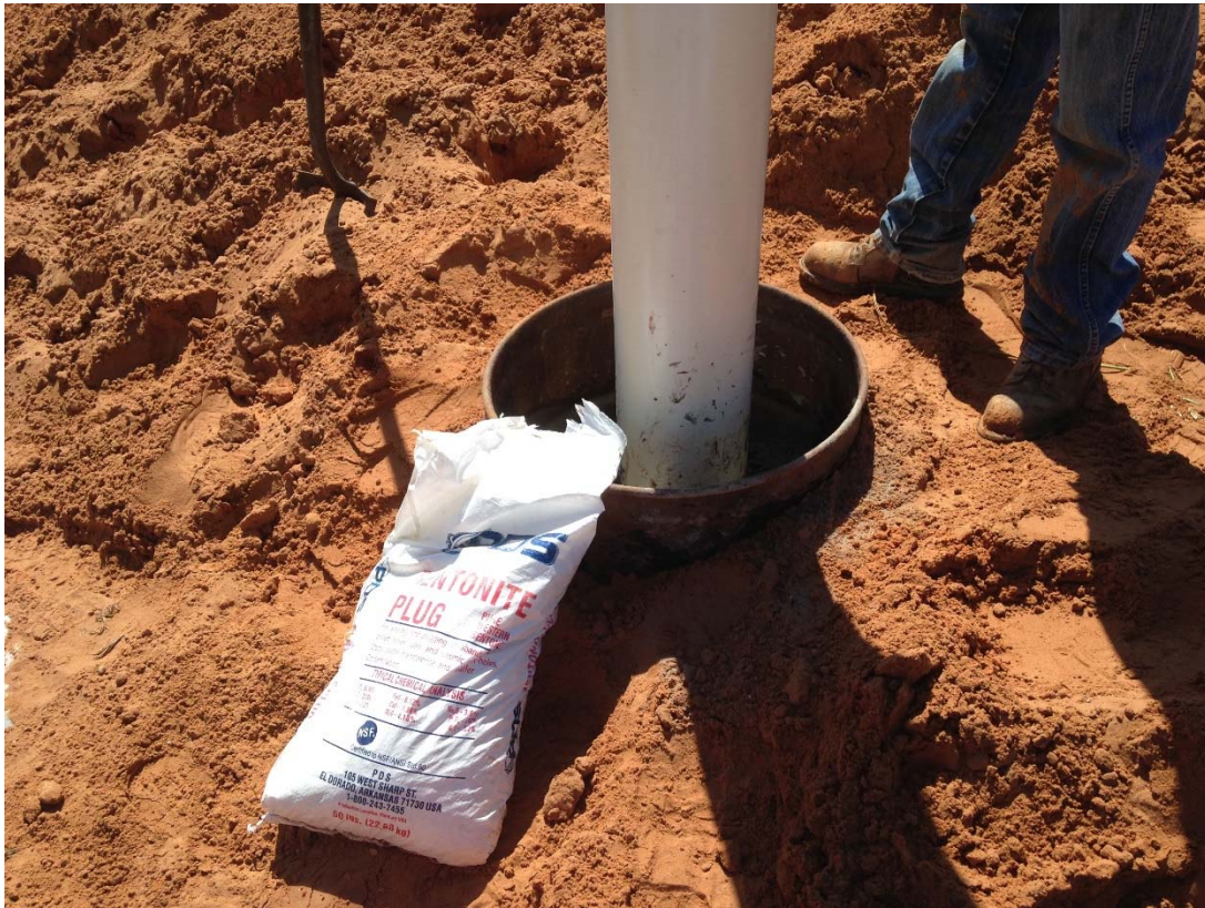
Photograph of the installation of 8" PVC casing conduits at the QPQASU #10 Flow Line Remediation Site.
