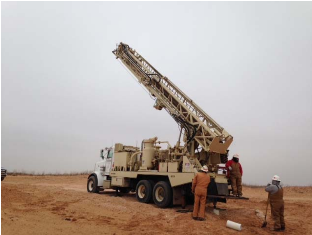
Photograph of soil boring activities at the QPQASU #10 Flow Line Remediation Site.
