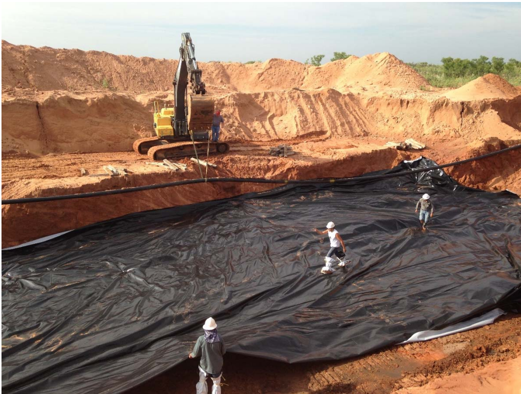
Photograph of the installation of an NMOCD-approved liner in the Eastern Release excavation at the QPQASU #10 Remediation Site.
