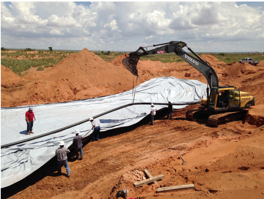
Photograph of the installation of an NMOCD-approved liner in the Western Release excavation at the QPQASU #10 Remediation Site.
