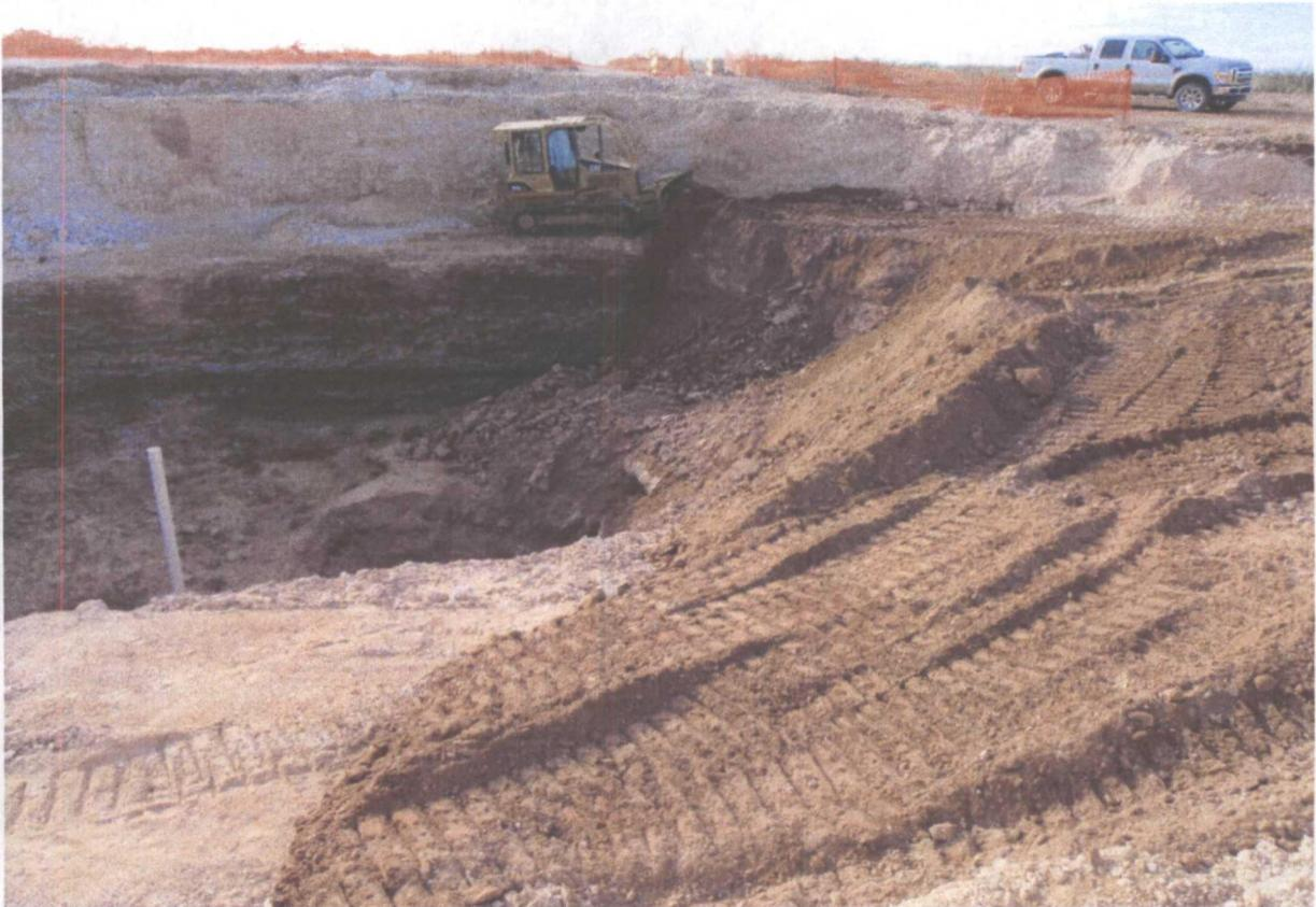
Photograph (looking East) of backfilling activities to allow for drilling at G.H. Cobb Federal #1.
