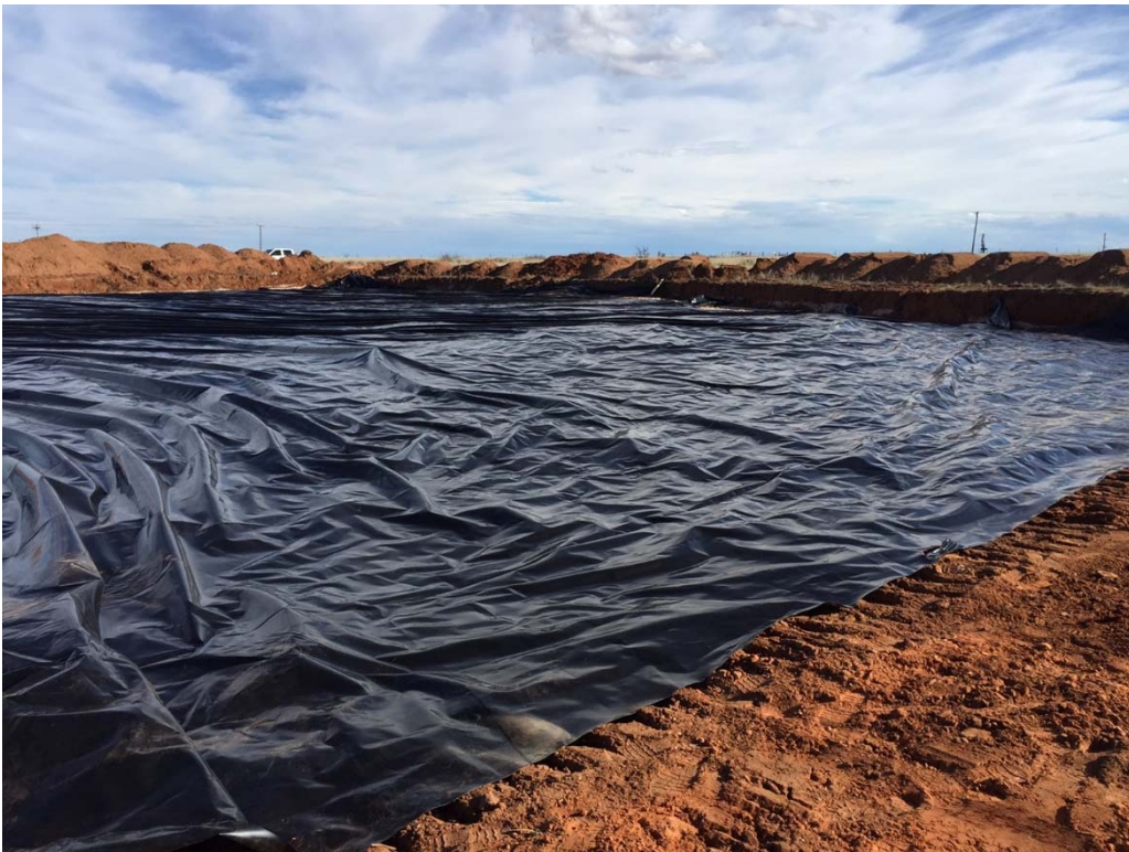
Photograph #2 – South liner installation
