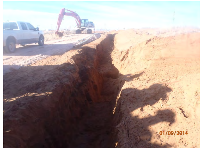
Excavation ready for liner, facing southwest
