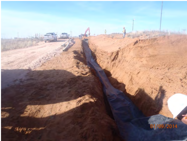
Installing liner in excavation, facing west 1/9/14
