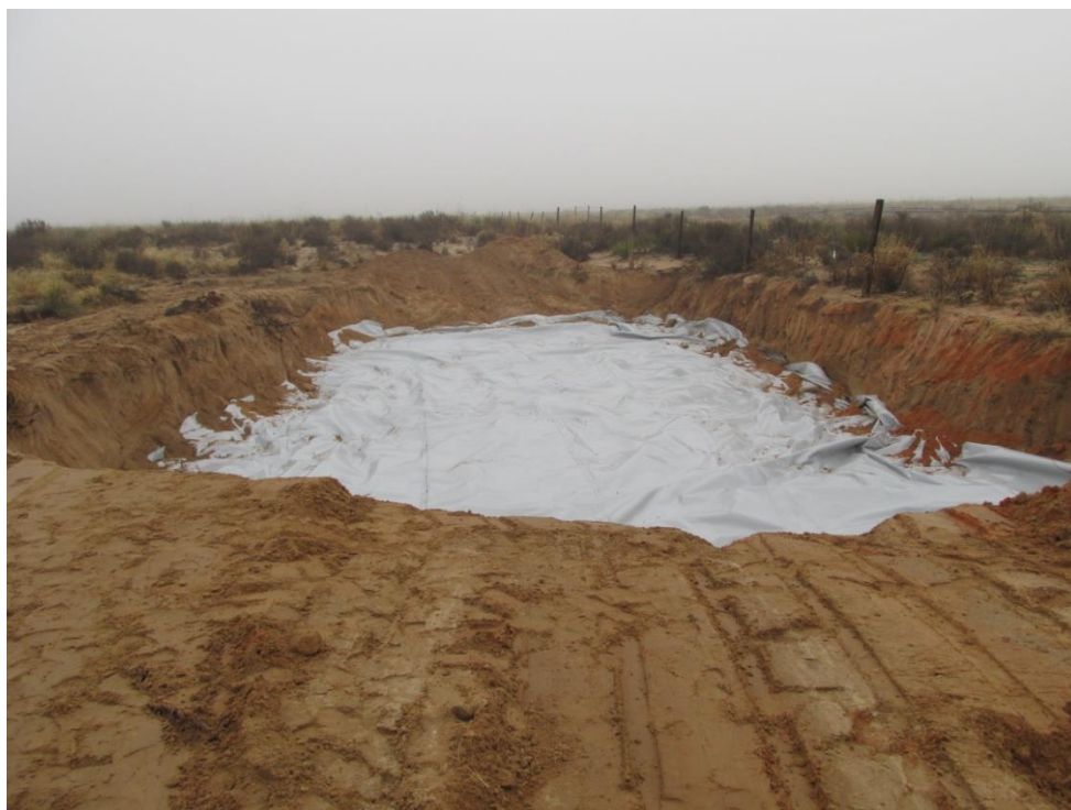
Photo 5 – Placement of liner and backfill of western release area.
