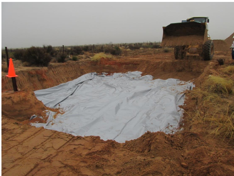
Photo 6 – Placement of liner and backfill around monitoring well of western release area.
