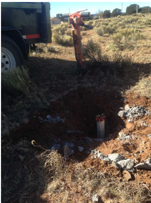
Photo 4. Photo facing southwest; of MW-5-41B following well pad removal.
