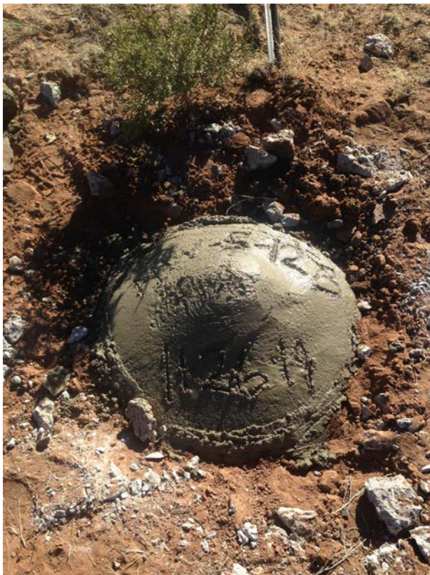
Photo 6. Photo facing south, of MW-5-12B plugged and abandoned.
