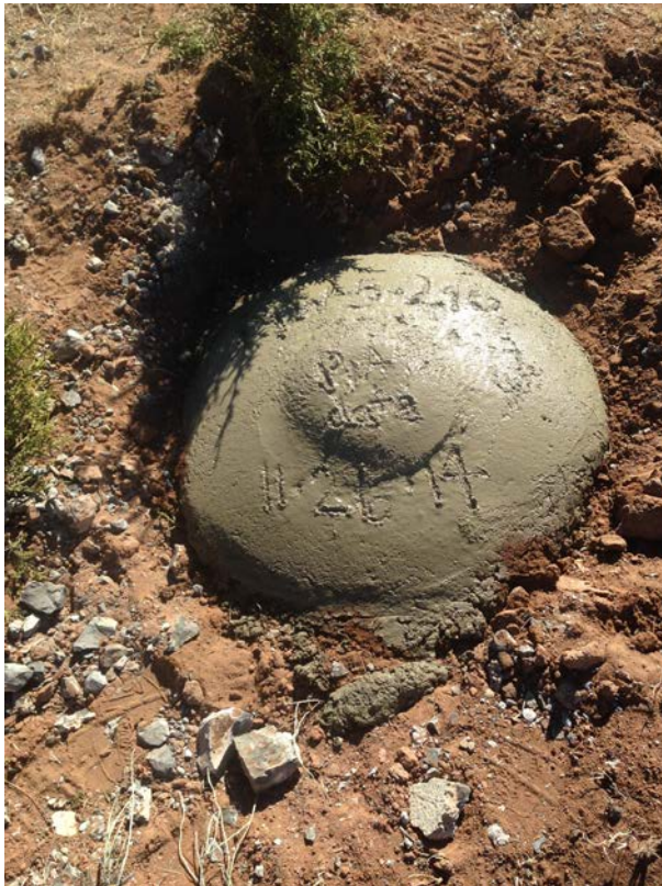
Photo 5. Photo facing south, of MW-5-24B plugged and abandoned.
