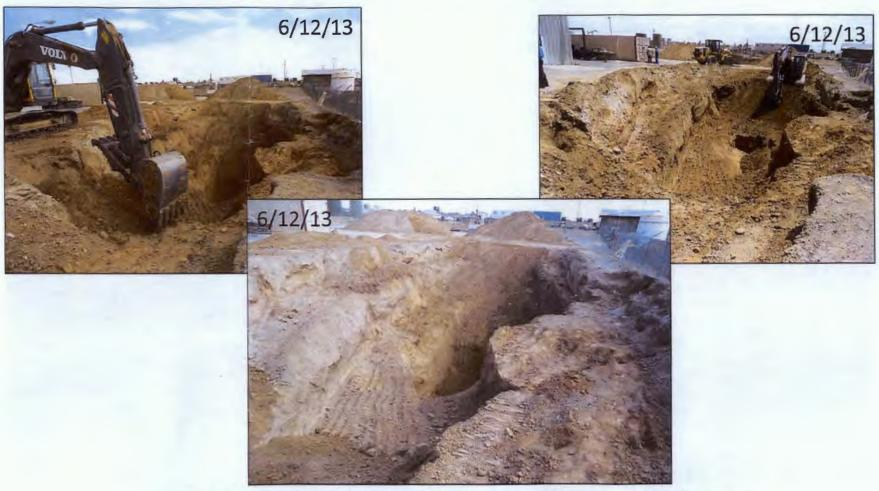
These photos facing south of the excavation show the benching that was required to extend the vertical reach of the excavator.
