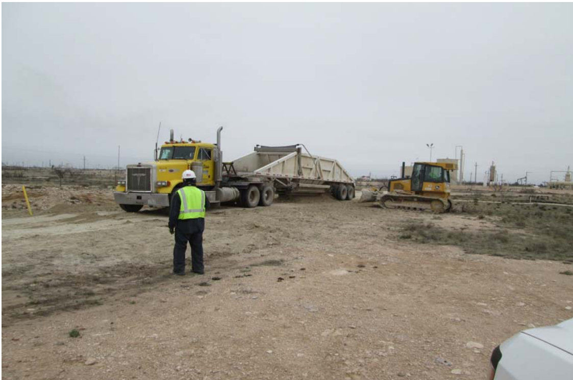
PHOTO 3: View of haul truck dispensing clean soil and heavy equipment facing west
