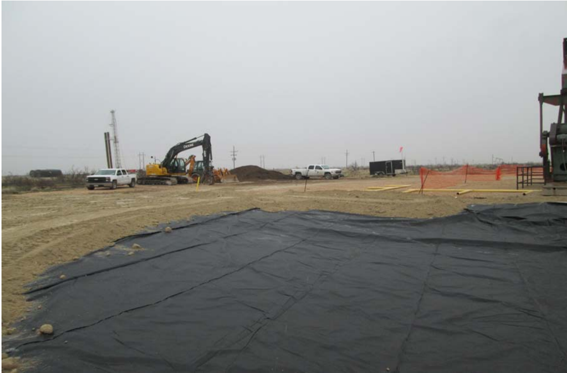
PHOTO 7: View 20-mil poly liner installation facing south
