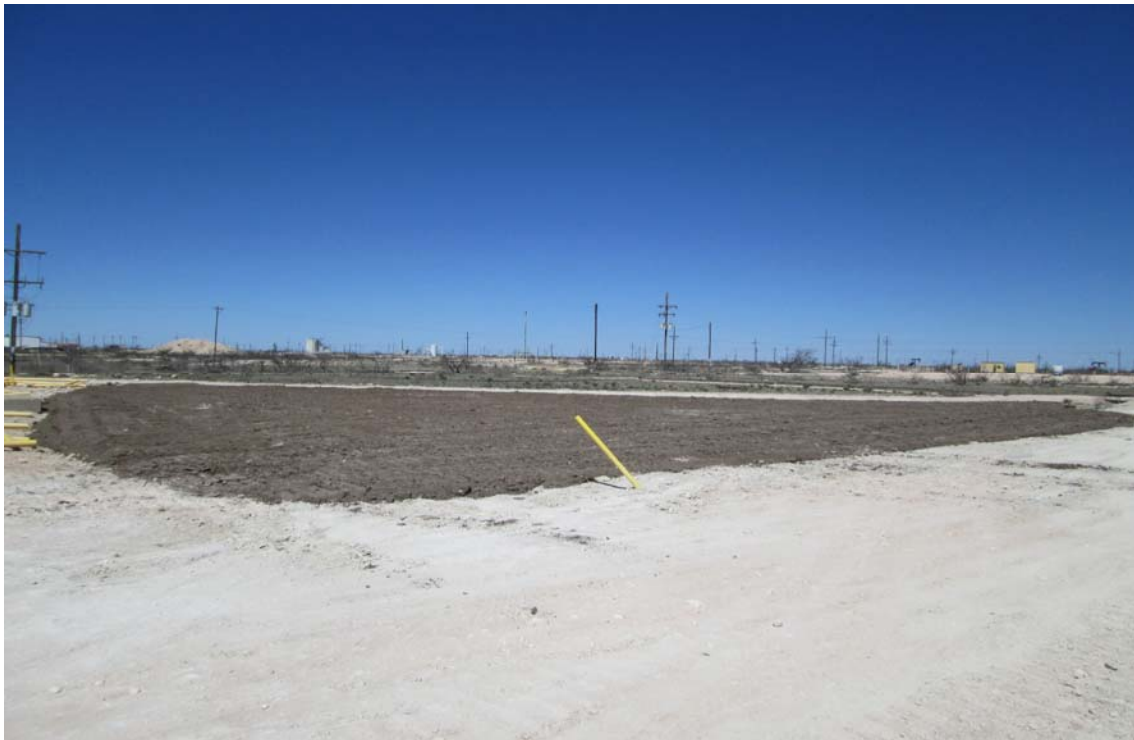
PHOTO 10: View of final grading, contouring, and seeding activities facing north west
