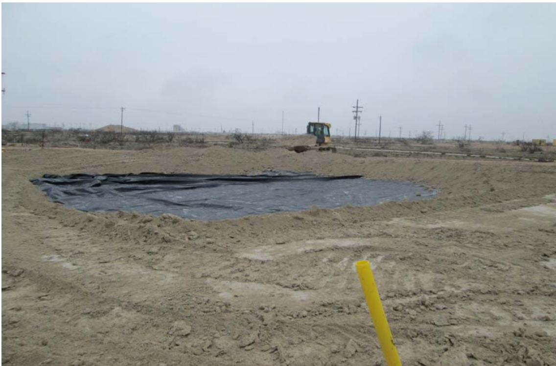
PHOTO 8: View of 20-mil poly liner installation and backfill activities facing north
