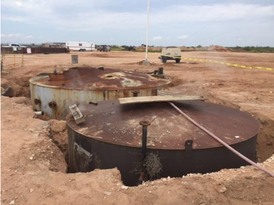
PHOTO 4: View of Classifier Tanks after de-piping, facing north.
