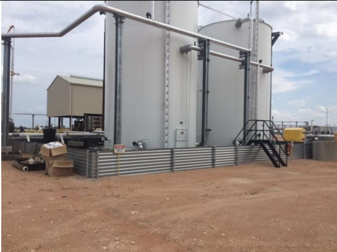
PHOTO 3: View of above ground storage tanks and associated containment built to replace Classifier Tanks, facing southeast.
