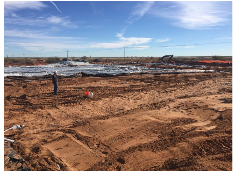
Photo 4: View of sampling area with plastic sheeting removed.
