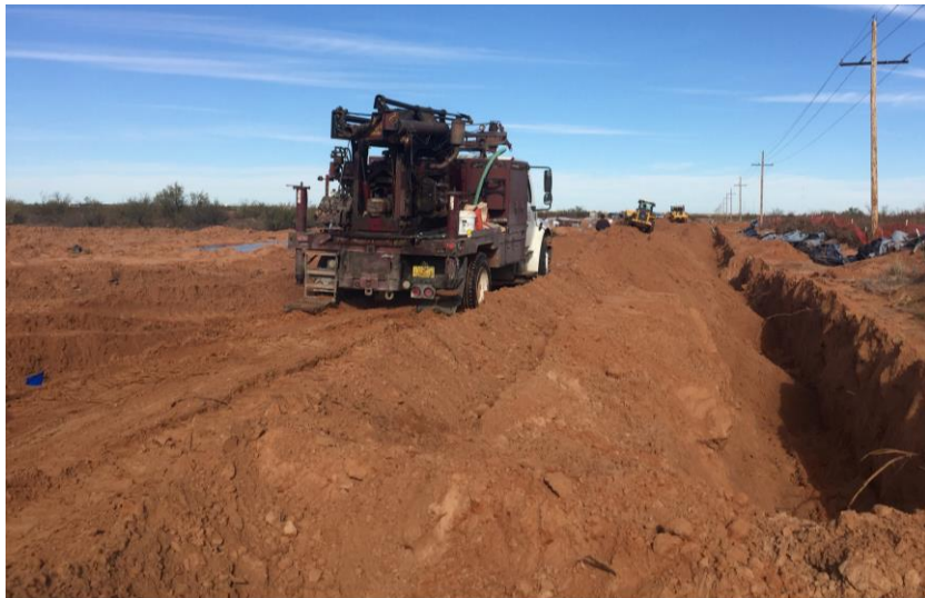
Photo 3: View of hollow stem auger CME rig mobilizing to next sampling location.
