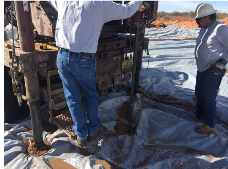
Photo 2: View of a typical boring installed via hollow stem auger CME rig on the plastic sheeting.
