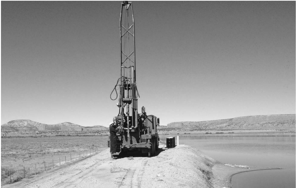
Set Up on Soil Boring SB-8N - Looking North
